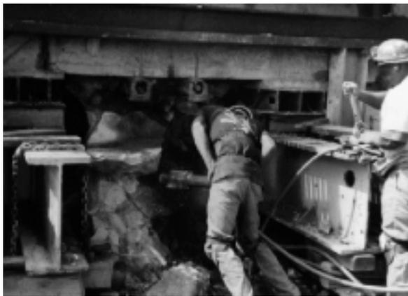
**Figure 19.** Once the initial lift was performed, the remaining foundation between the beams was removed.
