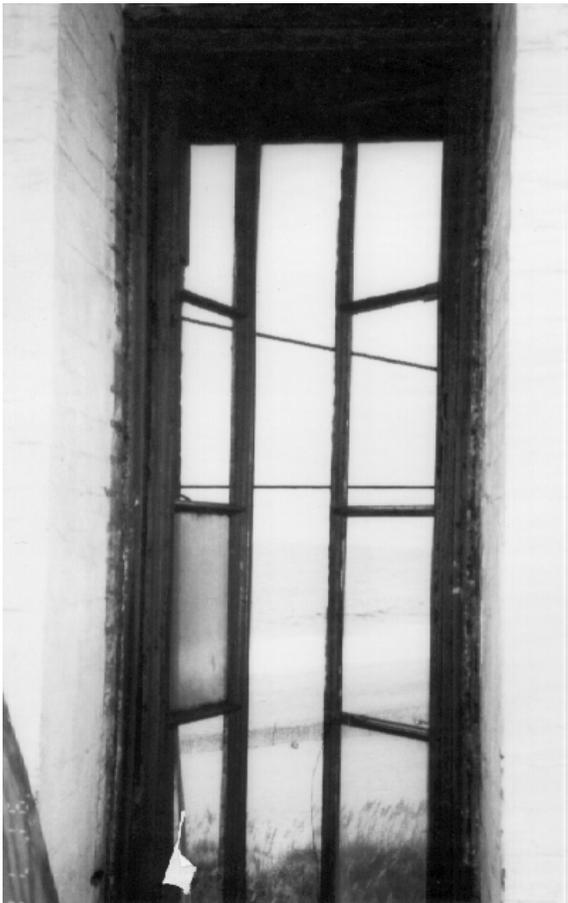
**Figure 11.** Example of a metal casement window in a lighthouse dating from the 1870s
