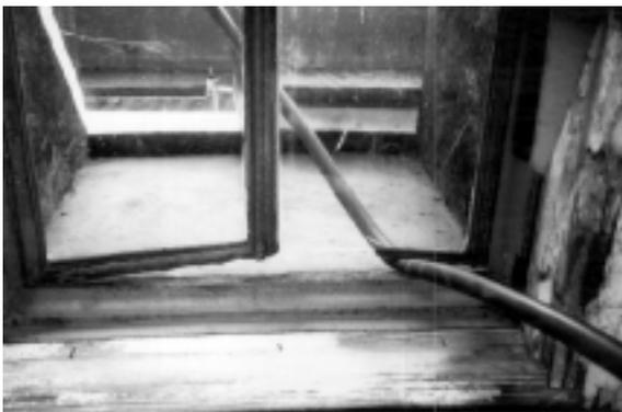
**Figure 12.** Close-up of severely deteriorated bottom rail of the same window in Figure 11. This condition can be repaired by splicing a new piece of sash
