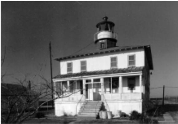
**Figure 2.** Example of a keeper's quarters fitted with a prefabricated cast-iron-and-steel lantern.
