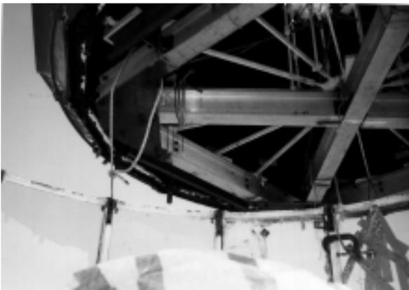
**Figure 5.** As the roof is being removed from the lighthouse, the tie rod system, supported by ICC's aluminum roofing frame, is visible. This frame was designed to fully support the roof and alleviate any stress or strain on the roof during the lift. Protruding down from the roof are the ends of the rafters which connect to the top of the stiles.
