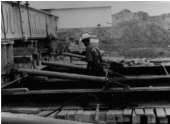
**Figure 20.** Four hydraulic rams set into the track steel pushed against the main steel to set the lighthouse in motion.
