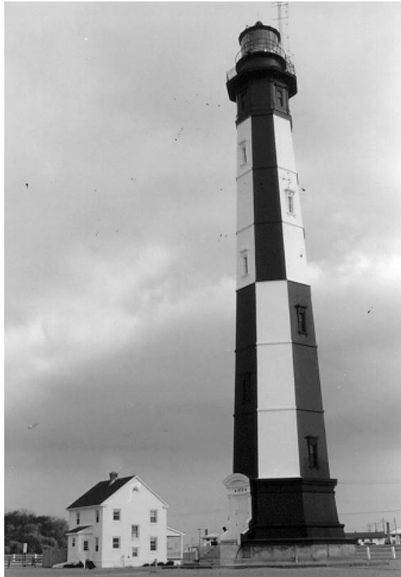
**Figure 4.** Double-wall, cast-iron, first-order 163-foot-tall coastal tower at Cape Henry, Virginia.
