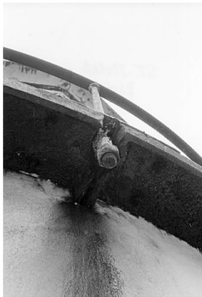
**Figure 10.** View of underside of gallery deck; the streaks on the stucco indicate that water is passing between the deck plates and possibly entering the masonry wall.
