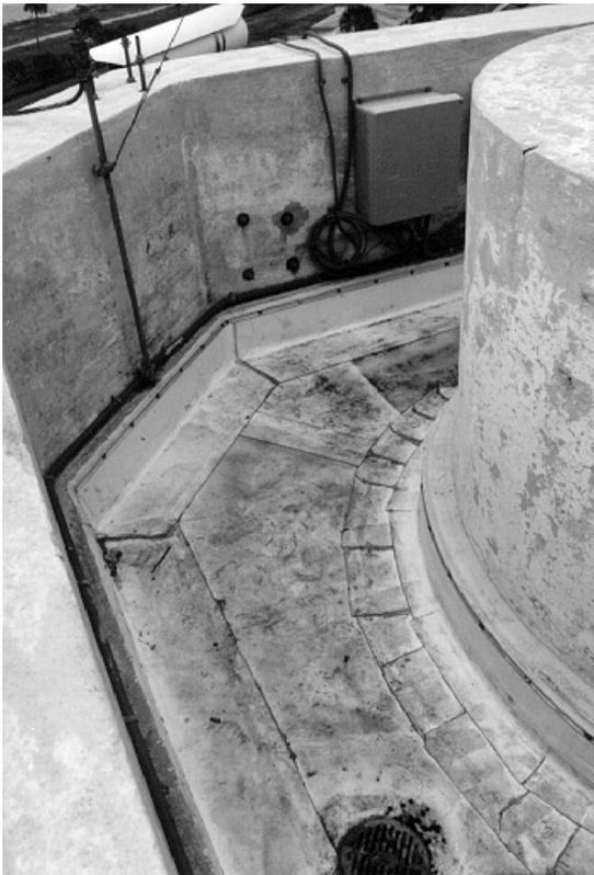
**Figure 7.** The concrete gallery deck on this concrete lighthouse has been covered with a rubber membrane. This covering should be checked regularly for leaks.
