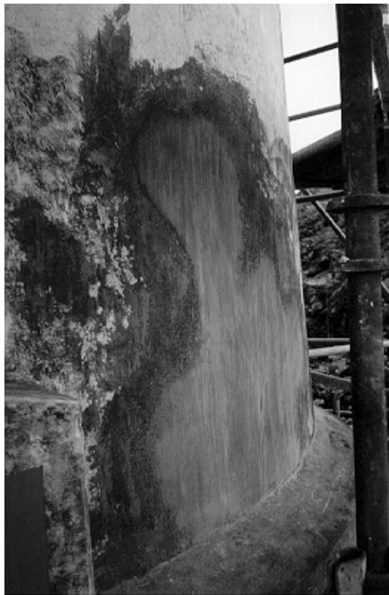
**Figure 27.** The areas where the loose mortar finish coat was removed were repaired with a two-part mortar patch. The final texture on the patch was tooled to match the historic wall surface. The patch was completely invisible after the tower was painted.
