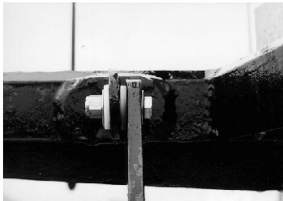
**Figure 25.** This is a view of a typical dissimilar metal isolation solution; the steel ladder post (vertical member in the center of the image) is isolated from the aluminum lantern gallery deck with nylon washers. The bolt chosen for this application is made from Type 316 stainless steel.
