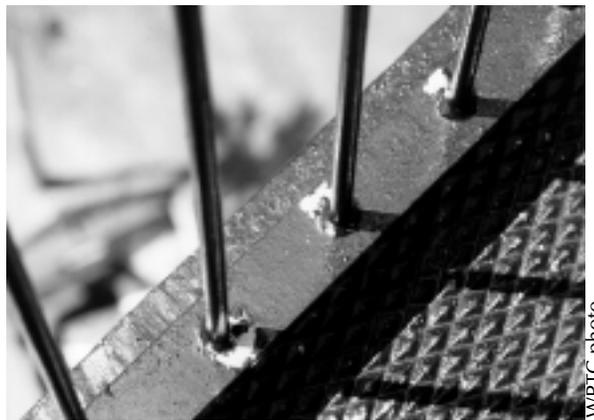
**Figure 40.** The paint on this stainless steel replacement gallery deck has begun to peel less than three months after it was painted. This could have been prevented if the stainless steel parts were first cleaned and then lightly glass-bead blasted.
