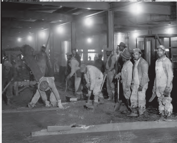
Workers pour and smooth the concrete floors inside K-25.
