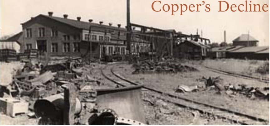
Materials and scrap parts lie around the idle C&H Foundry.
