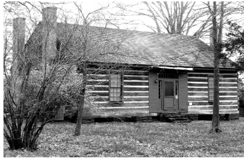
Kolb Farmhouse, post-restoration
