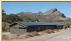
Pinnacles National Monument uses solar panels to power some of its facilities. In the Pacific West Region, over 700,000 kilowatt-hours of power were produced in 2008 from renewable sources.
