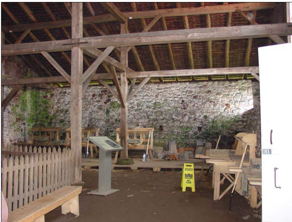
Figure 115. Interior north side of the cast house, view looking north, July 2006.
