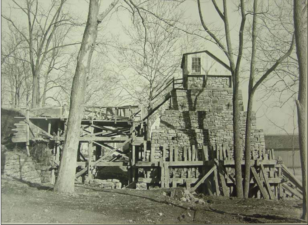
Figure 32. West elevation of the furnace, January 6, 1939.
