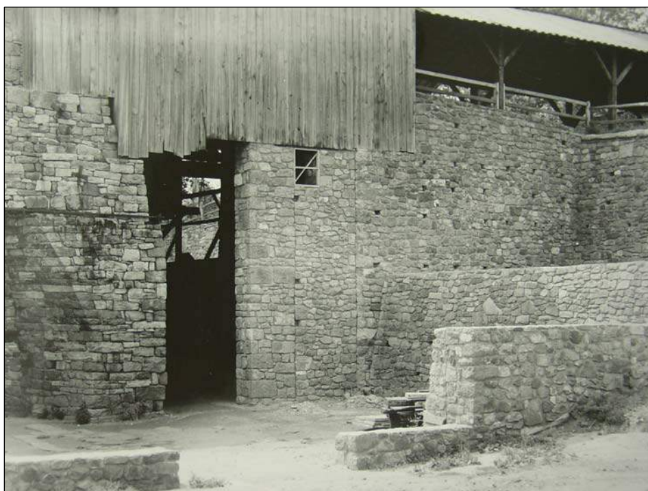
Figure 59. Partially rebuilt west wall of the cast house, north of the furnace, September 1963. The new wall is left of window below the bridge house.
