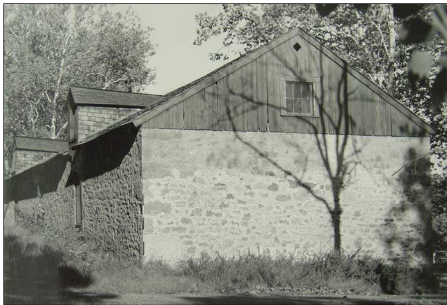
Figure 48. West and north elevations of the charcoal house, October 1956.
