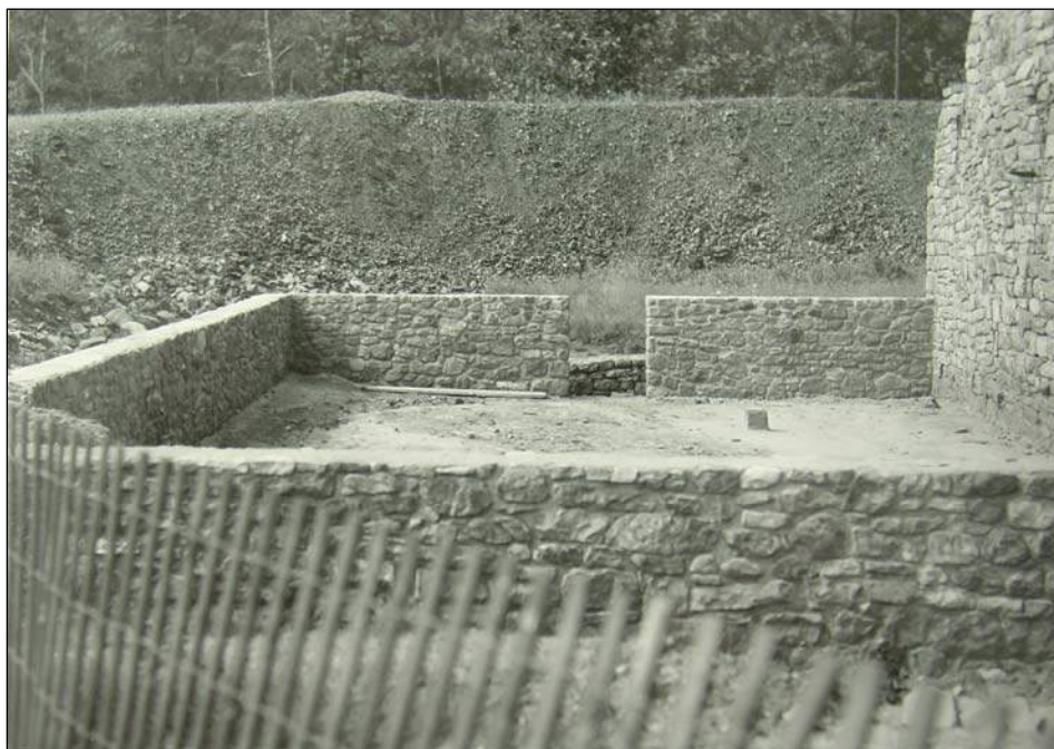
Figure 58. Rebuilt stone foundation walls of the cast house, south of the furnace, October 1962.
