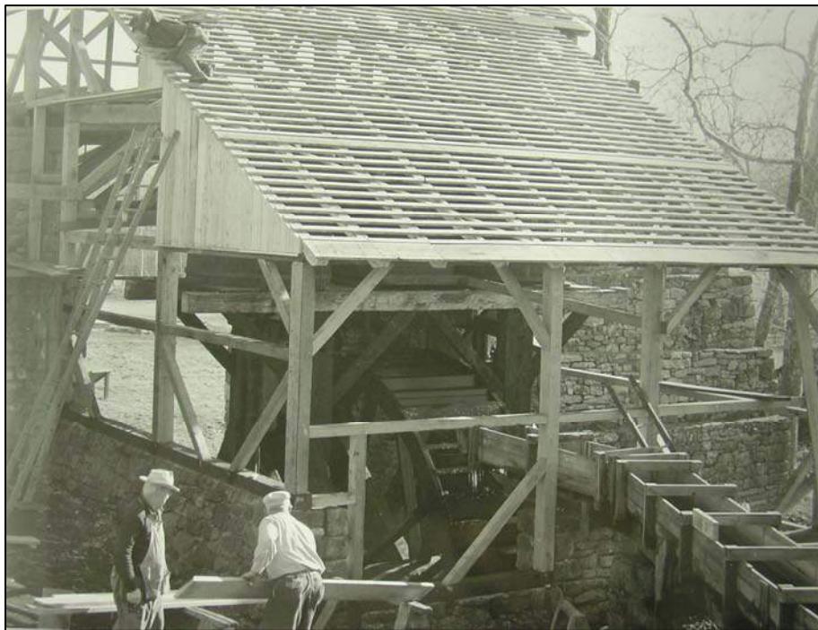
Figure 50. Reconstruction of the wheel house, November 7, 1957.
