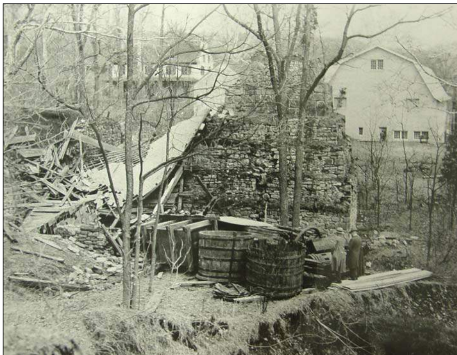
Figure 25. Final collapse of the wheel house and bridge house following removal of the water wheel and blast machinery (in foreground) by the Franklin Institute of Philadelphia in 1931.
