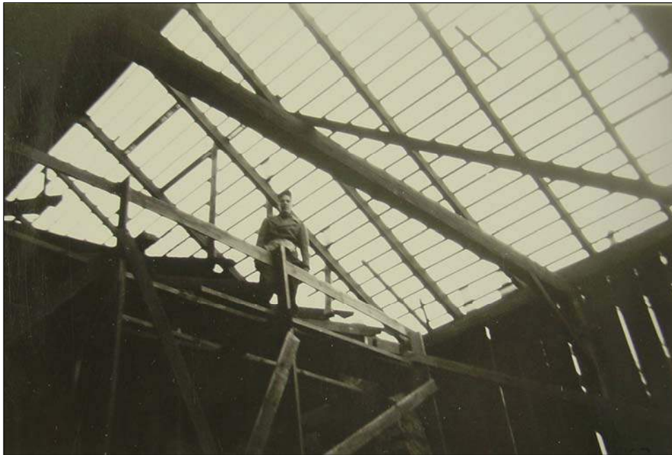
Figure 38. Reshingling of the charcoal house roof, December 1947.
