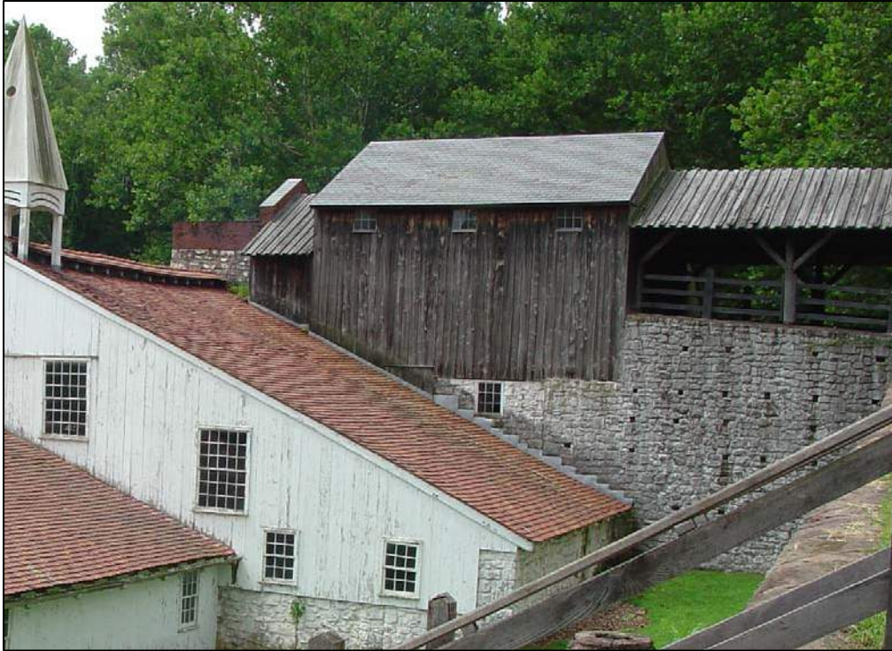
Figure 87. East elevation of the connecting shed, bridge house, and tunnel- head vestibule, July 2006.
