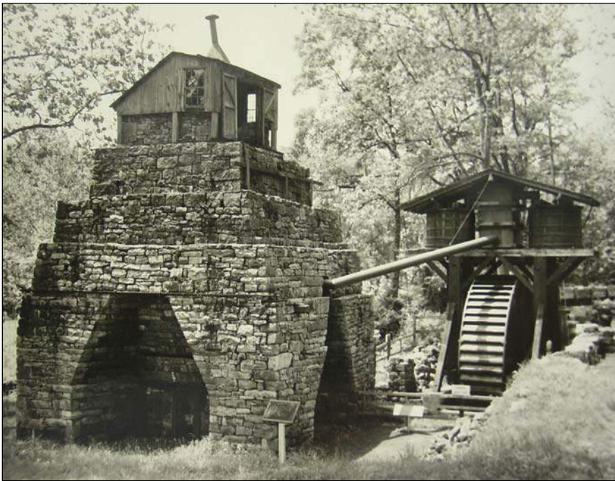
Figure 44. The completed water wheel and blast machinery with temporary roof, June 25, 1952. Note that the furnace walkway had been removed for this project and was not reinstalled.
