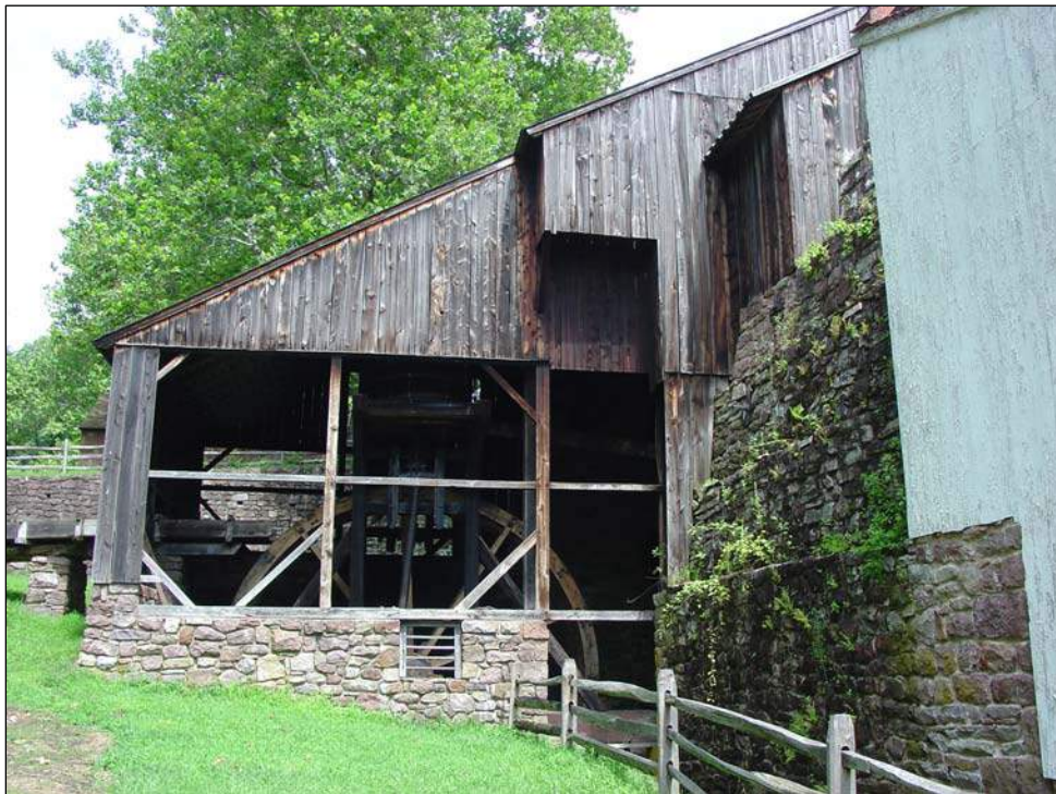
Figure 102. South elevation of the wheel house, July 2006.
