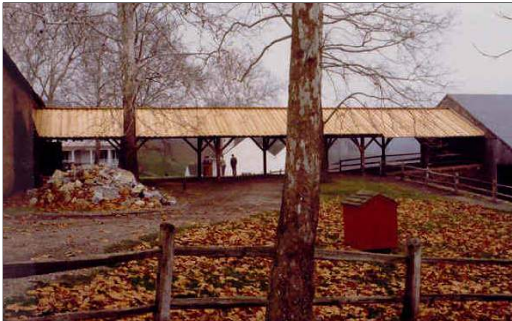
Figure 70. New roof on the connecting shed, Nov. 11, 1977.
