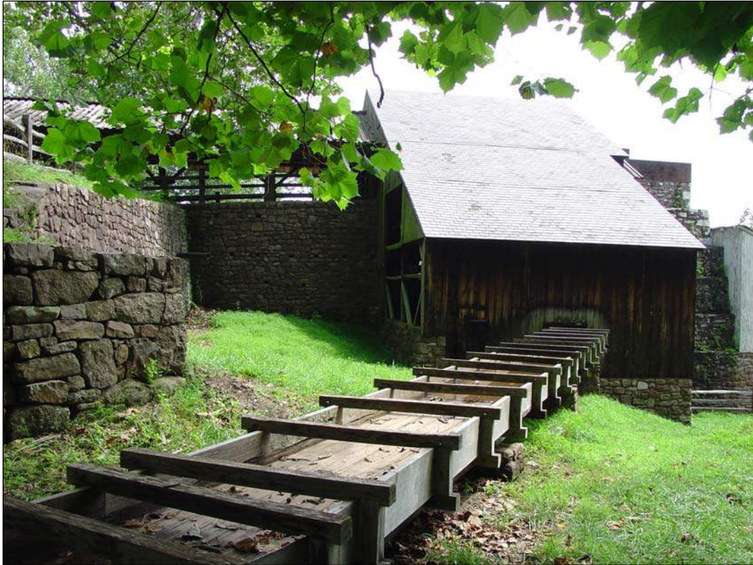
Figure 107. Flume of the west head race, view looking east towards the wheel house, July 2006.
