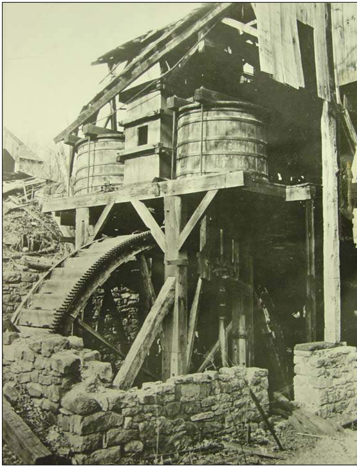
Figure 23. Appearance of the water wheel and blast machinery following the collapse of the wheel-house roof, 1926. Note the cogs on the side of the wheel that were probably installed at the same time as the steam engine in 1881.
