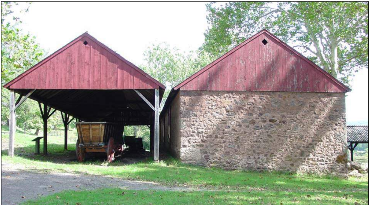
Figure 97. West elevations of the charcoal house (right) and cooling shed (left), September 2006.
