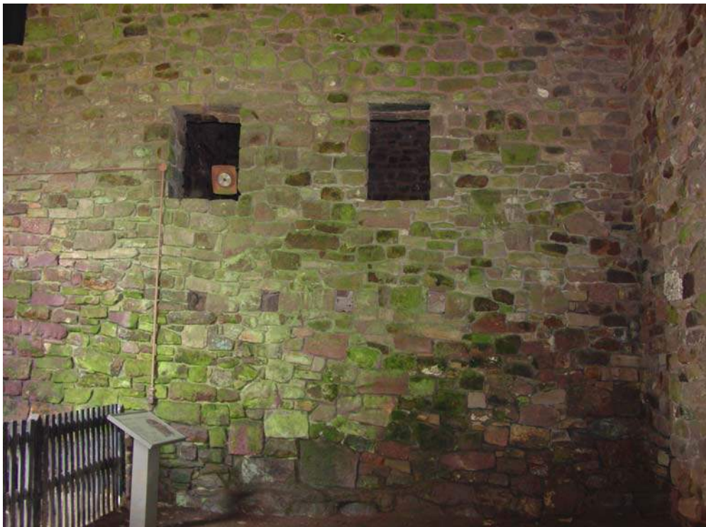
Figure 94. Reconstructed north wall ("Wall A") supporting the north end of the enclosed bridge house, July 2006.
