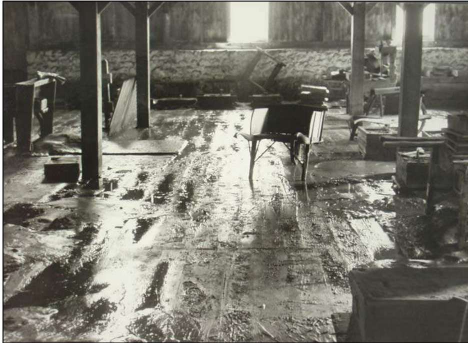
Figure 73. Post- hurricane damage in the cast house, 1987.
