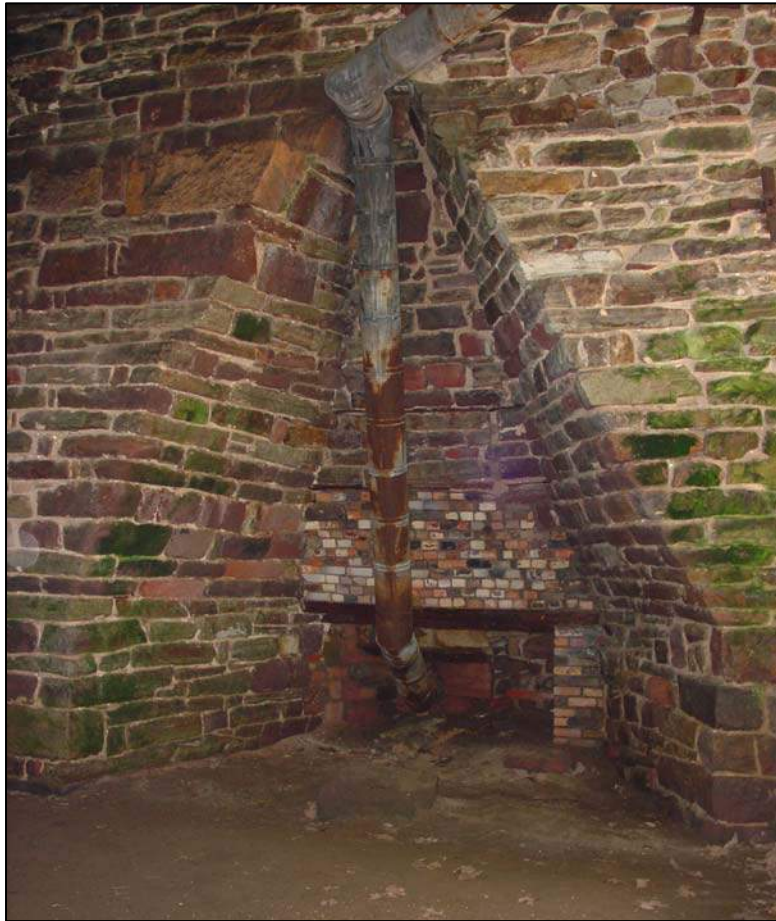
Figure 81. Tuyere arch on the north side of the furnace, July 2006.
