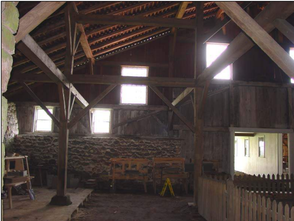
Figure 114. Interior north side of the cast house, view looking east, July 2006.
