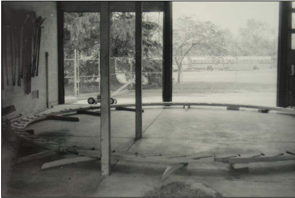
Figure 71. Construction of new water wheel, May 30, 1978.
