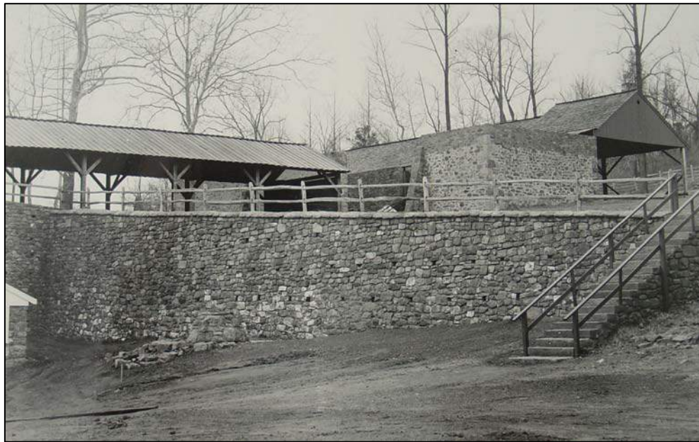
Figure 65. South and east elevations of the charcoal house following demolition of the roof and south extension, June 1965.
