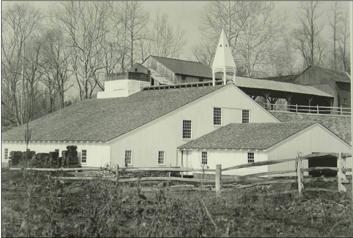
Figure 63. The completed cast house and east shed, March 29, 1965.
