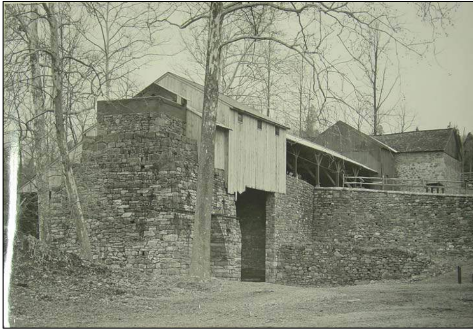
Figure 51. View of the Furnace Group from the southeast, showing the reconstructed bridge and wheel houses, March 4, 1958.
