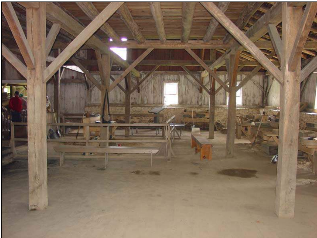
Figure 117. Interior south side of the cast house, view looking east, July 2006.
