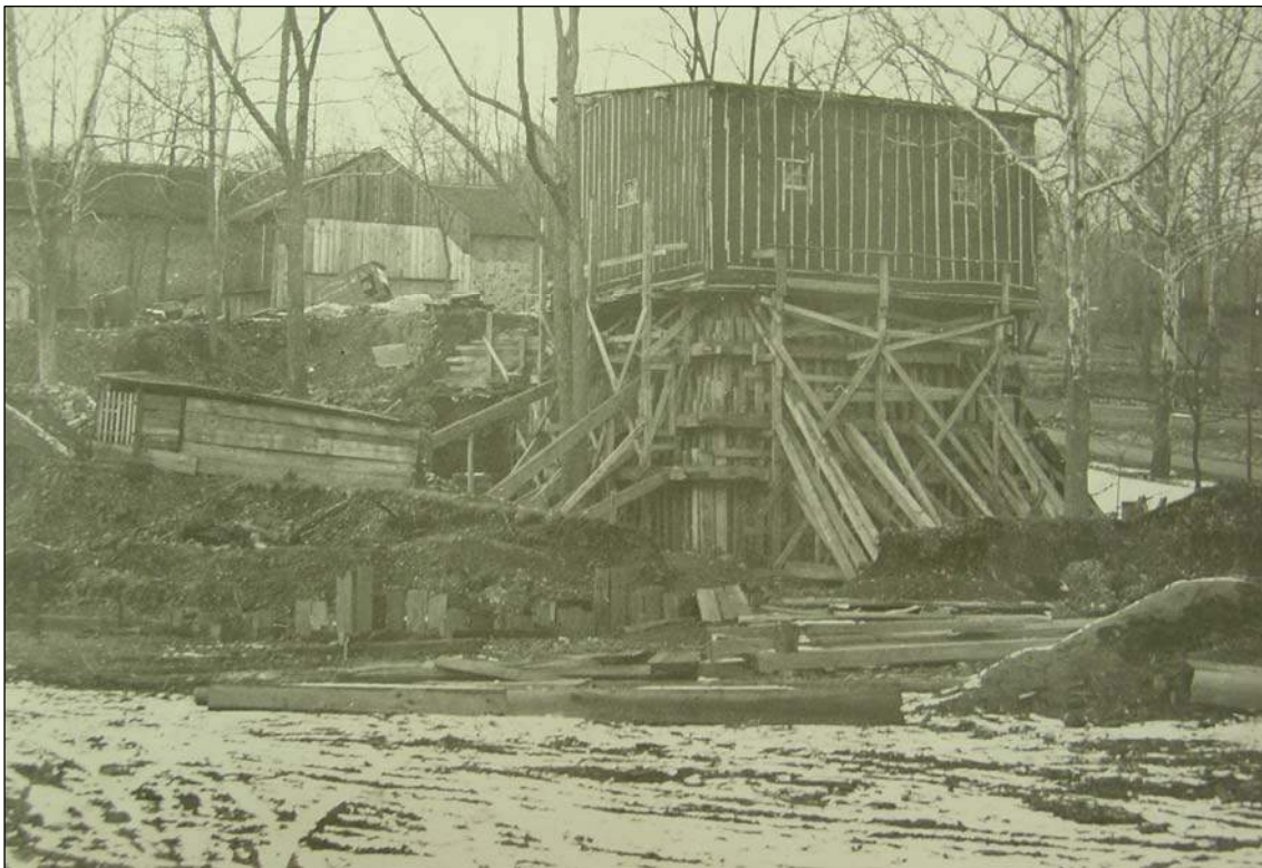
Figure 31. View looking northeast towards the charcoal house, showing temporary construction shed erected on top of the furnace stack, February 26, 1937.
