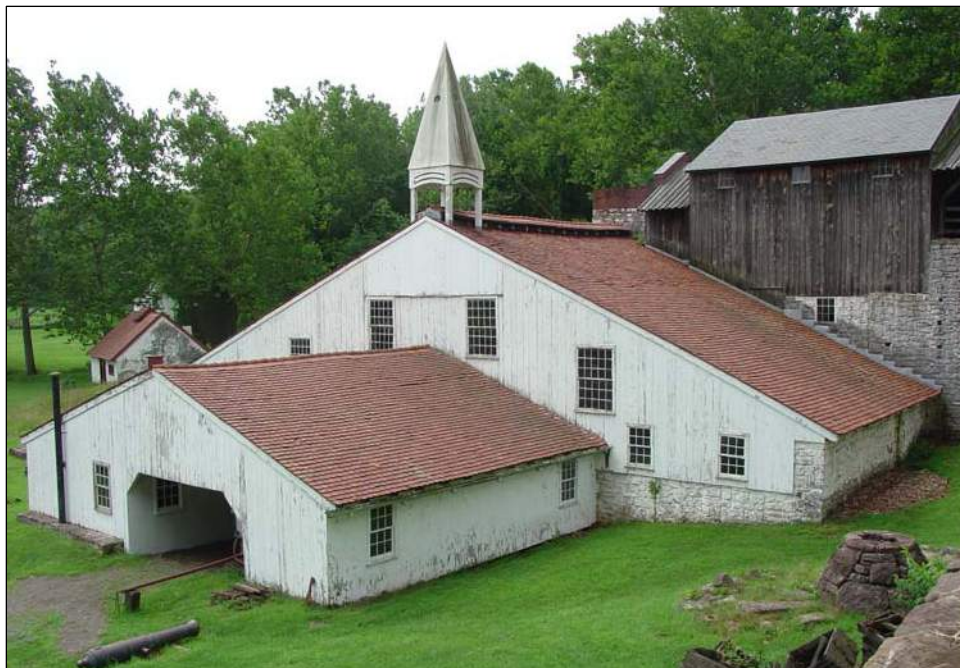
Figure 111. North and east elevations of the cast house and east shed, July 2006.
