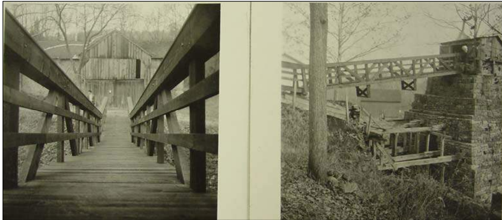
Figure 39. New “temporary” furnace walkway, November 7, 1947.
