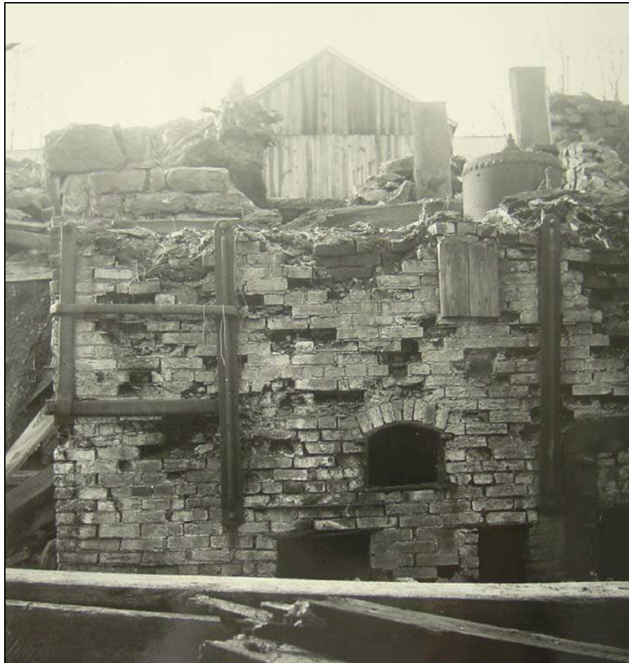
Figure 41. South brick wall enclosing the steam boiler prior to dismantling, 1950. Note also the south extension of the charcoal house in the background.
