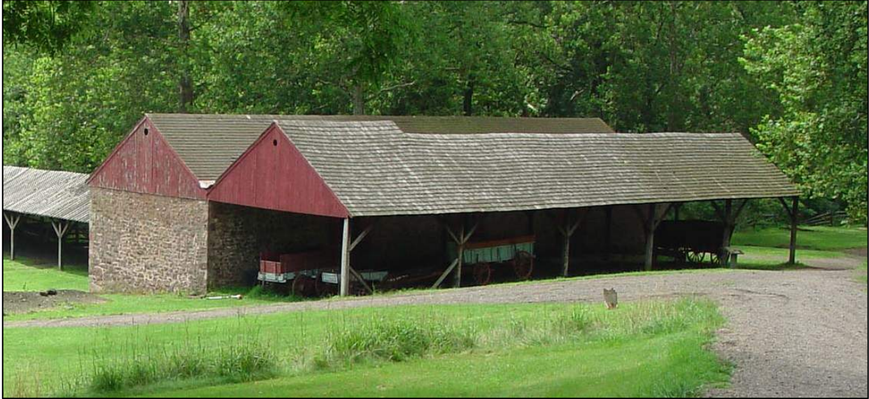
Figure 96. North and east elevations of the charcoal house and cooling shed, July 2006.
