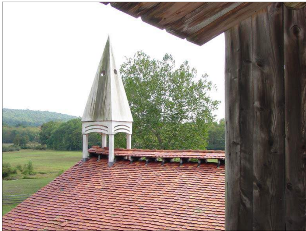
Figure 113. Detail of the cast house roof and belfry, September 2006.
