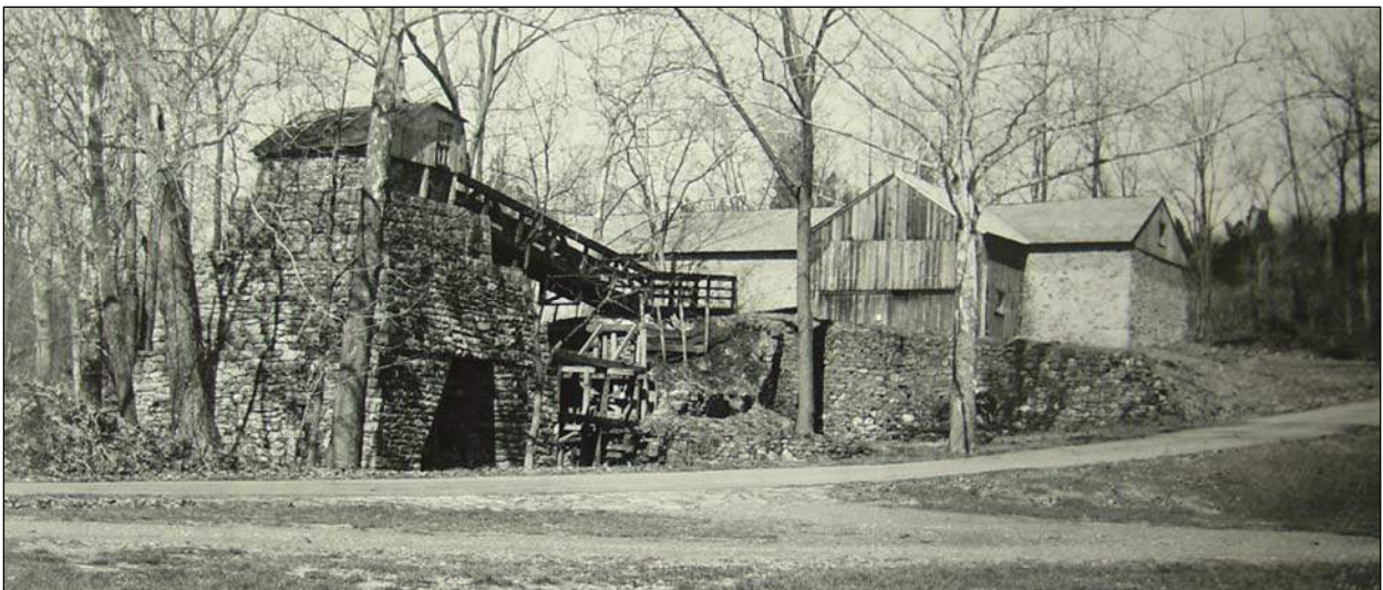
Figure 40. General view of the Furnace Group with new furnace walkway, as seen from the southeast, April 17, 1948.
