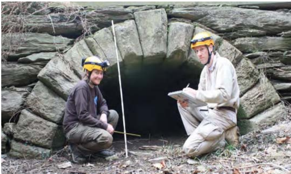
Exploring the Tailrace Tunnel, Harpers Ferry NHP
