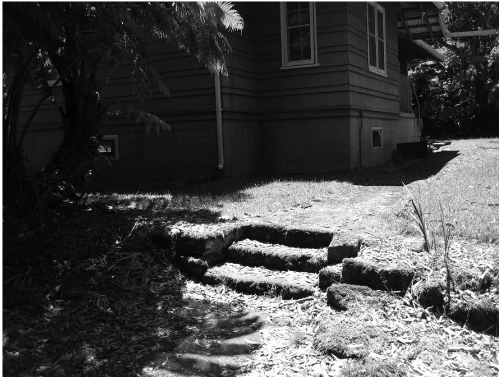
Figure 5. Example of mortared lava stairs and footpath leading from carport to backdoor of residence (PWR Staff—2005).
