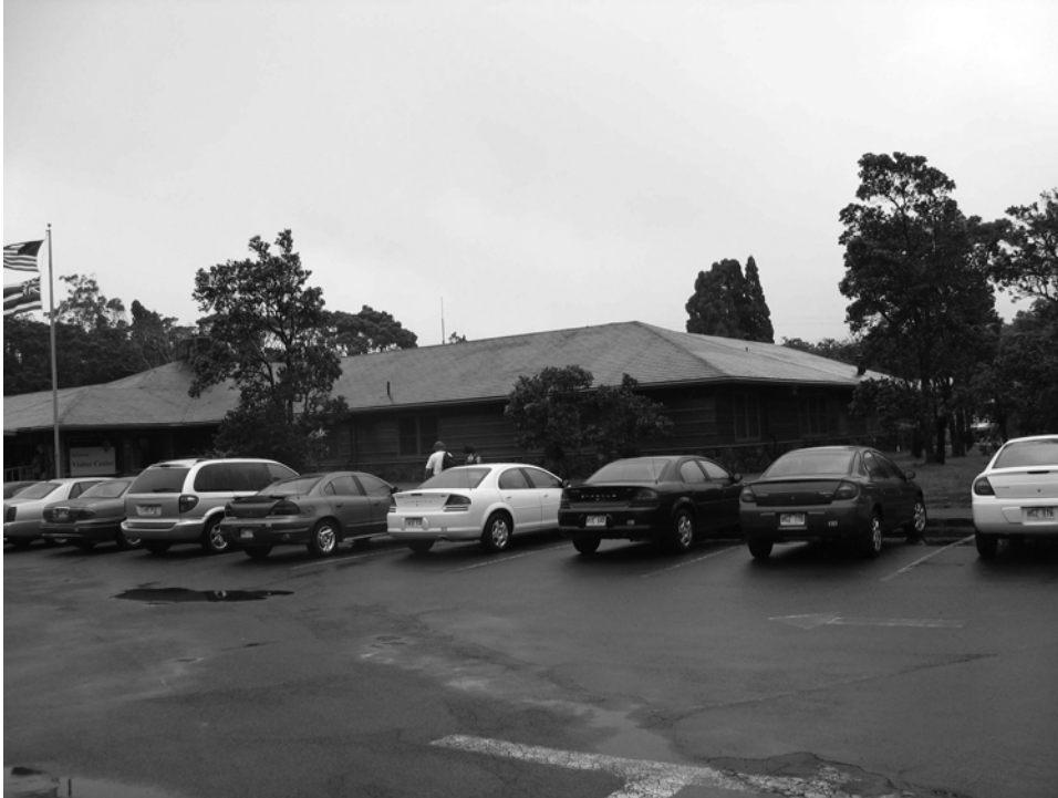
Figure 6. Current view of Administration Building (PWR Staff—2005).
