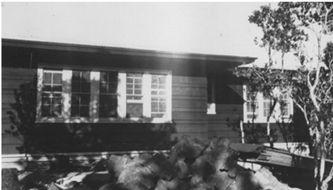
Figure 1. Employee Residence being built (1945 NPS Travelogue, HAVO Archives).
