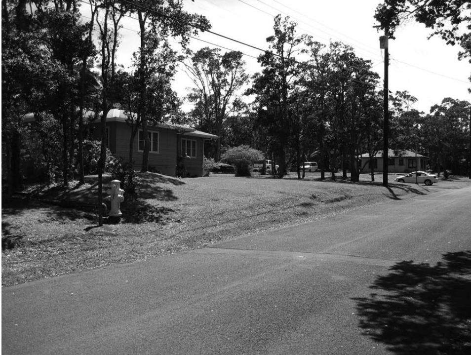
Figure 3. Lots were graded to create boundaries between the units—Employee Quarters No. 19 (PWR Staff—2005).
