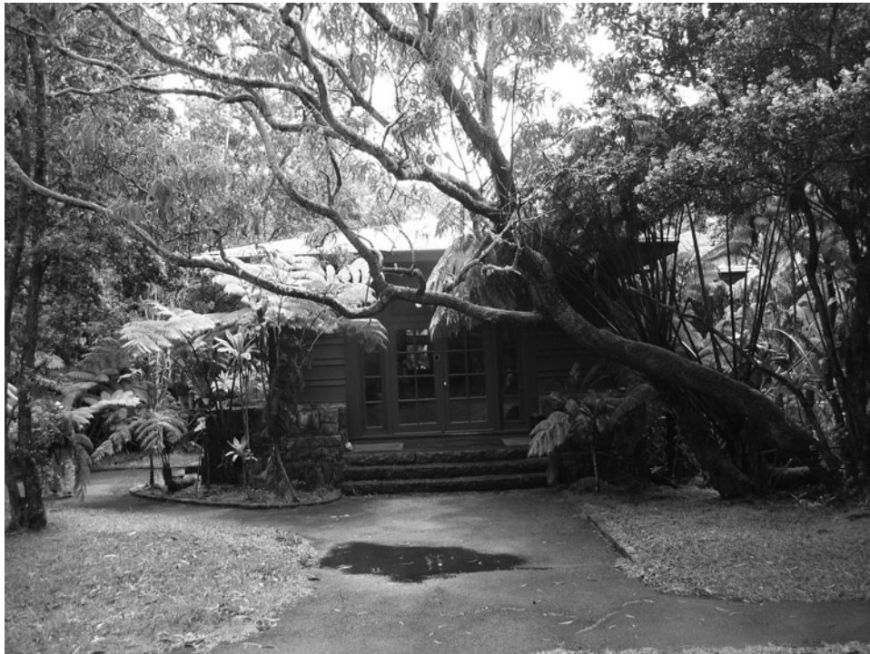
Figure 7. South entrance of the Ohia Wing (PWR Staff—2005).
