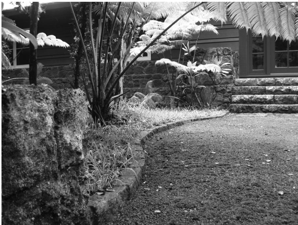
Figure 6. Stone curbing, wall and stairs at north entrance of the Ohia Wing (PWR Staff—2005).
