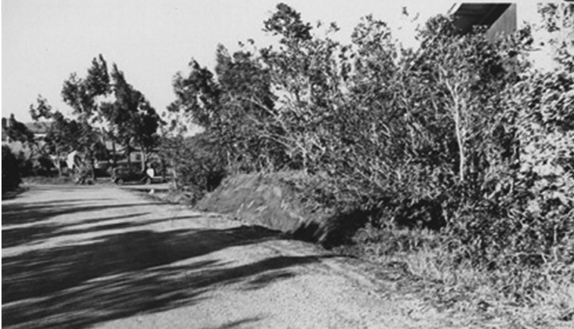
Figure 1. Photograph from the 1939 landscape architect report showing rounding of road banks (1939 Landscape Architect Report, HAVO Archives).
