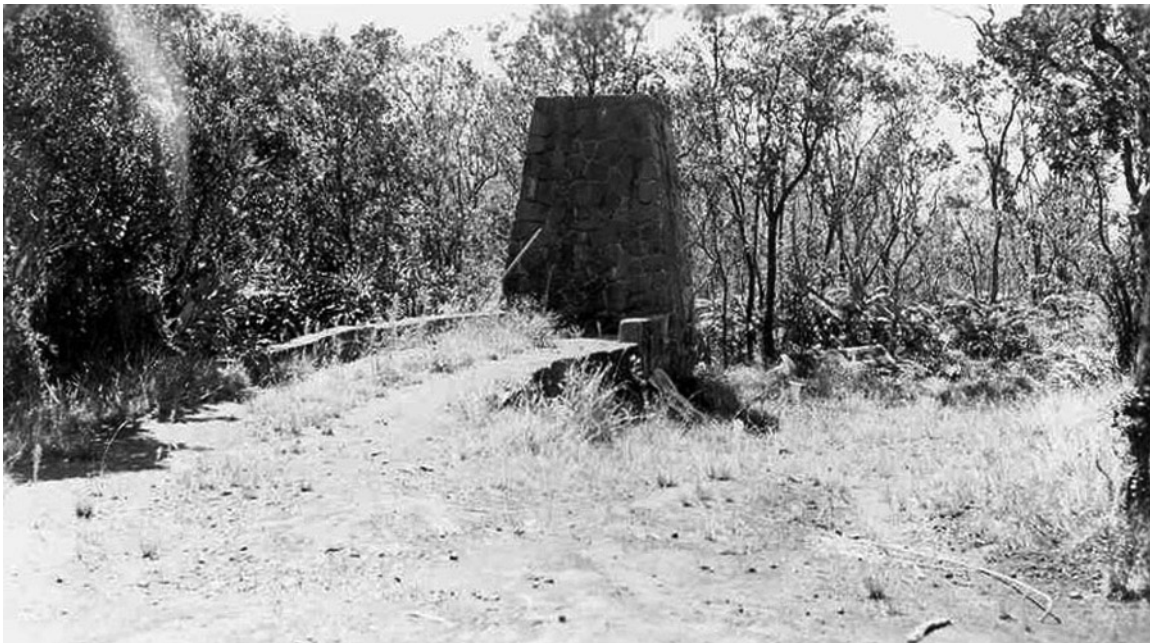
Figure 9. Abandoned incinerator located between CCC camp and NPS employee housing area. (PWR Staff—2005).
