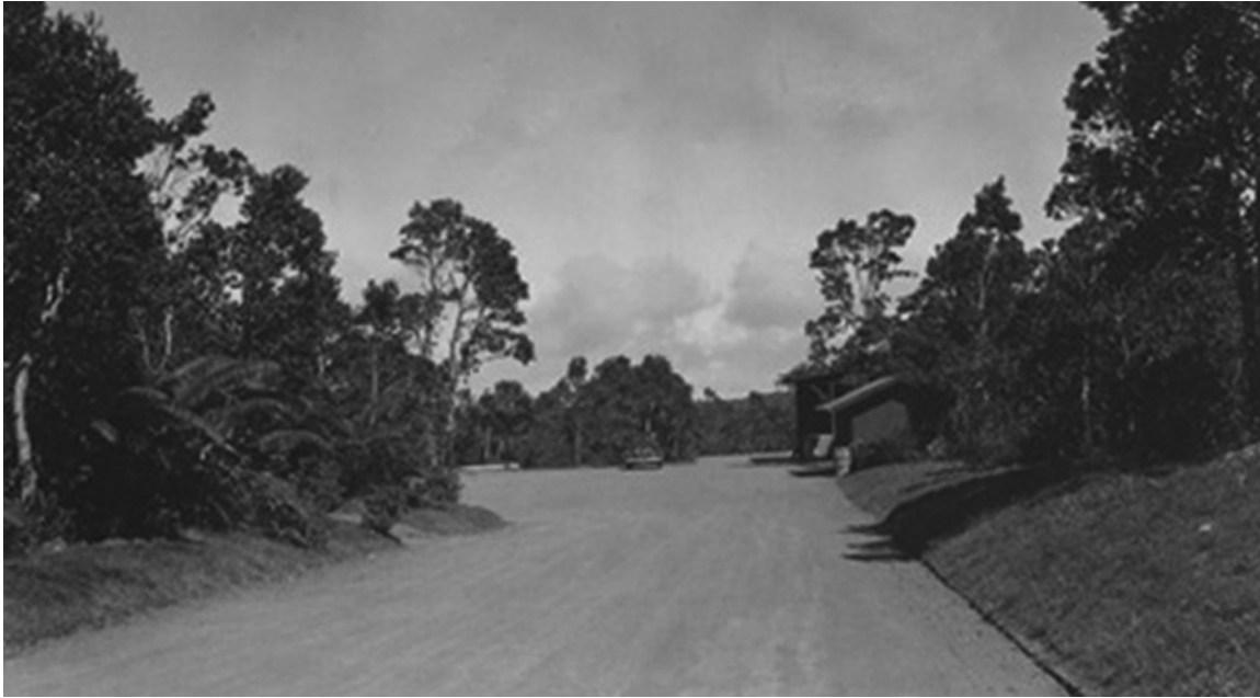
Figure 1. Main Residential/Maintenance Area Road facing maintenance area. Photo taken after surfacing was completed and shoulders were sloped and graded (1934 Landscape Architect Report, HAVO Archives).
