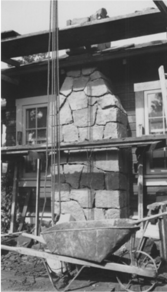
Figure 3. Stone chimney being added to Employee Quarters No. 5 in 1934—six years after the residence was built (1934 Landscape Architect Report, HAVO Archives).
