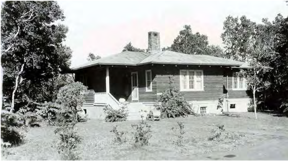
Figure 2. Example of a typical residence (Employee Quarters No. 22) ca. 1945, approximately six years after it was built. The building was designed to blend in with the surrounding native vegetation. (1945 NPS Travelogue, HAVO Archives).
