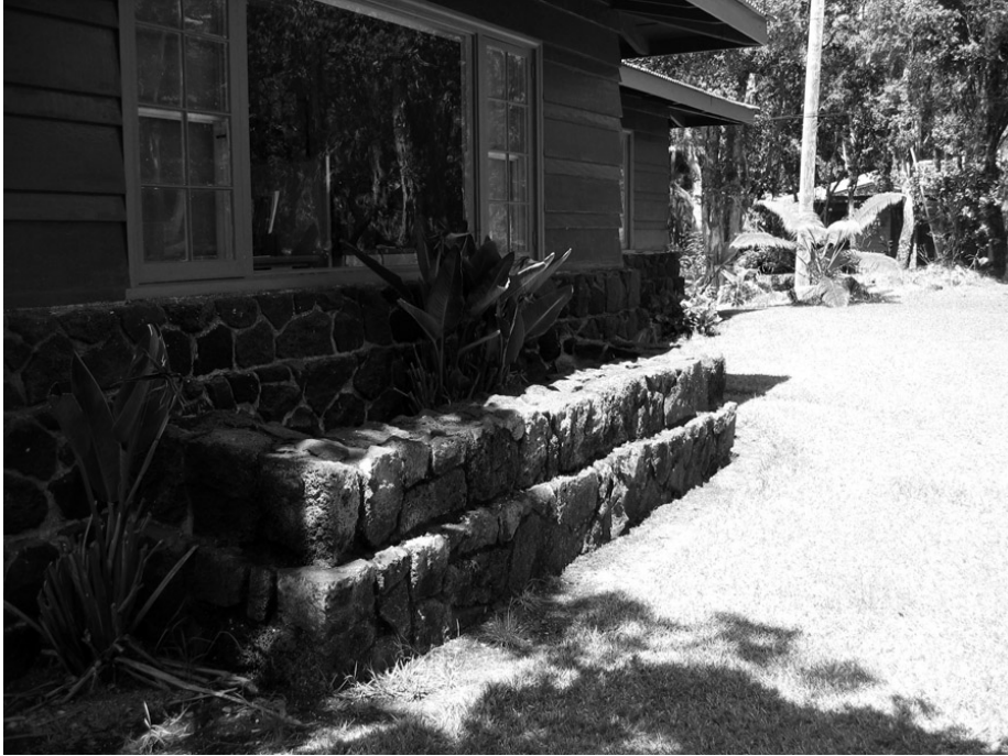
Figure 1. Example of a mortared lava-rock planter in employee housing area (PWR Staff—2005).
