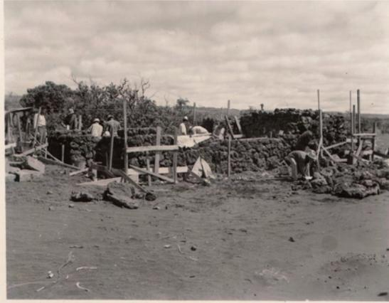
2 views of Footprint Museum shelter under construction by CCC (job B-19). Building is to provide shelter for visitors while viewing footprints which will be enclosed in concrete and glass case. Materials donated by Hui O Pele.
