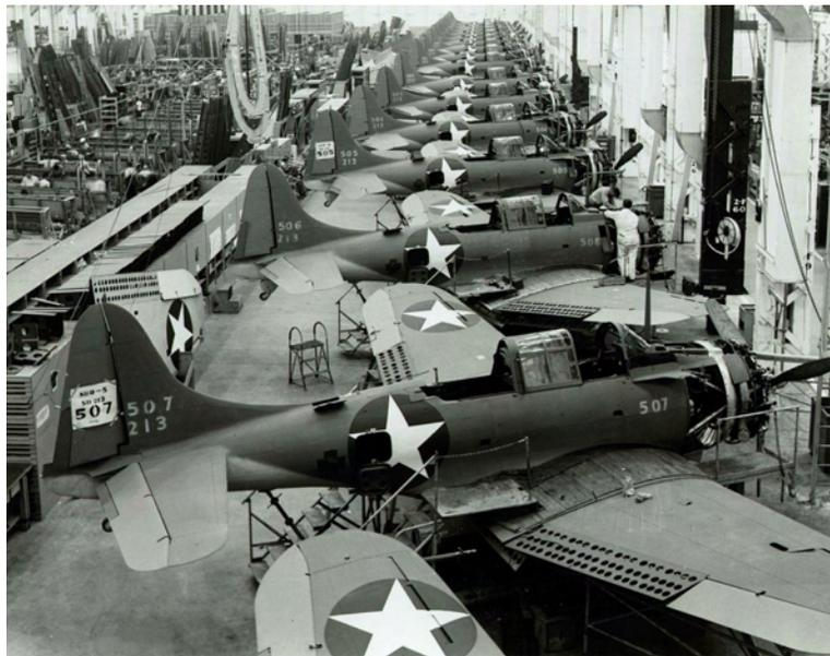
**6. 8. Douglas SBD Dauntless manufacture, El Segundo Plant, California, 1942. The Corsair (Vought F4U) would soon replace the Dauntless as the US Navy's fighter plane of choice.**
