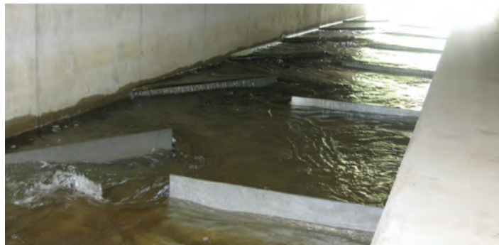
Ditch Creek highway culvert is outfitted with baffles to aid fish swimming upstream by giving them spots to rest out of the main current.
