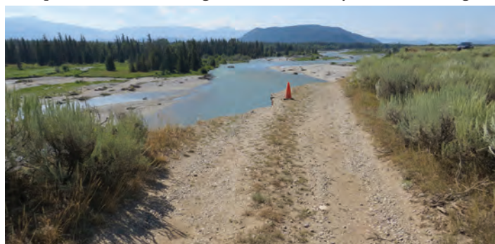
The River Road is no longer passable due to bank erosion along the Snake River, and was closed permanently as outlined in the Wild and Scenic River Plan.
