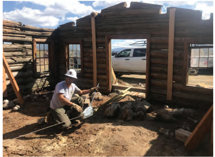
A preservationist cinches the cable brace used to hold the structure together while stabilization work is done on the deteriorating main Bar BC cabin.
