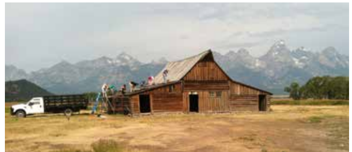
Volunteers replacing the roof on the TA Moulton Barn on Mormon Row.
