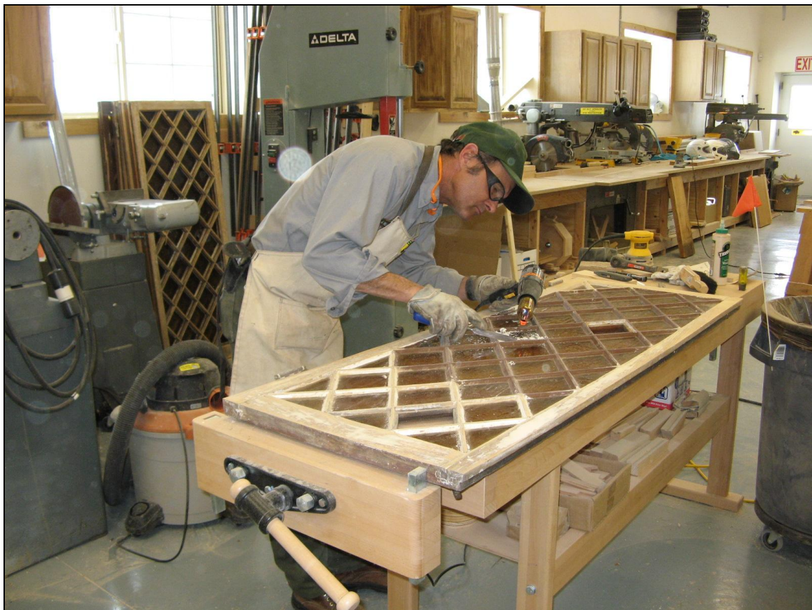
Figure 6: Al Williams, WCHP, stripping existing paint from windows.
