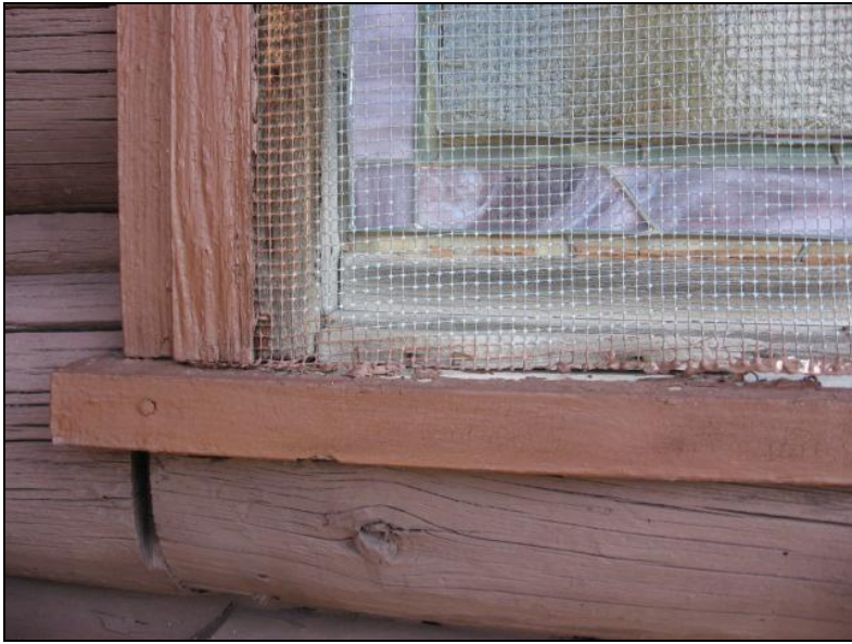
Figure 4: Insufficient mesh & distressed sill.
