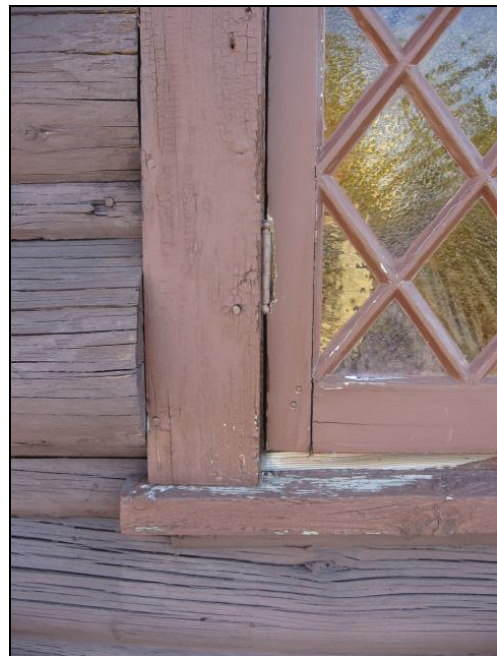
Figure 3: Unpainted, cracked, and rotting sills and framework.
