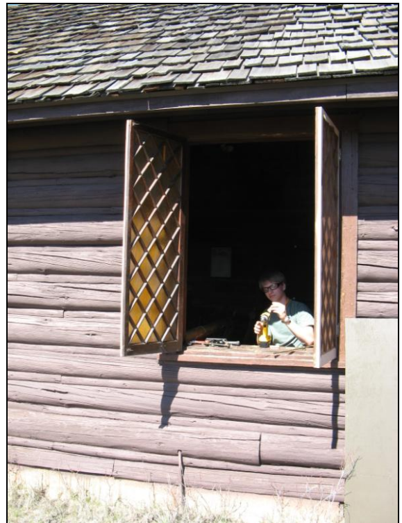
Figure 10: David Stubbs, WCHP, reinstalling paned window sashes into their framing.
