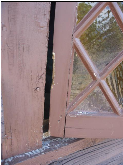
Figure 2: Missing hardware that was causing further damage to framing and sills.
