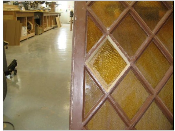
Figures 7 & 8: Replacement and reglazing of similarly colored glass pane.
