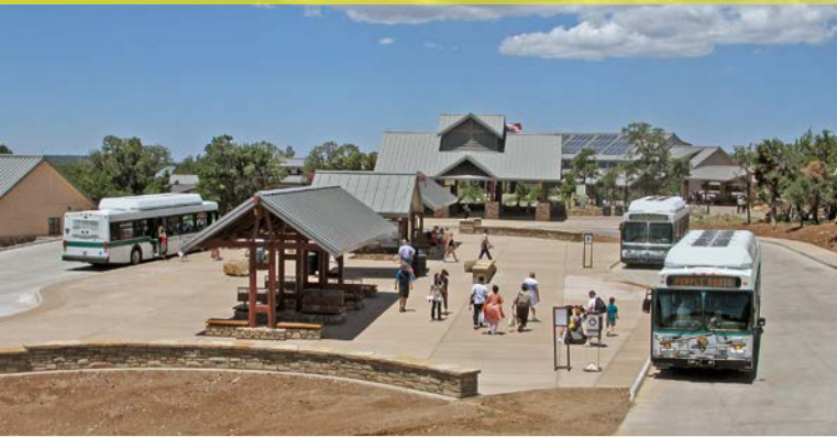
Grand Canyon Visitor Center Complex
