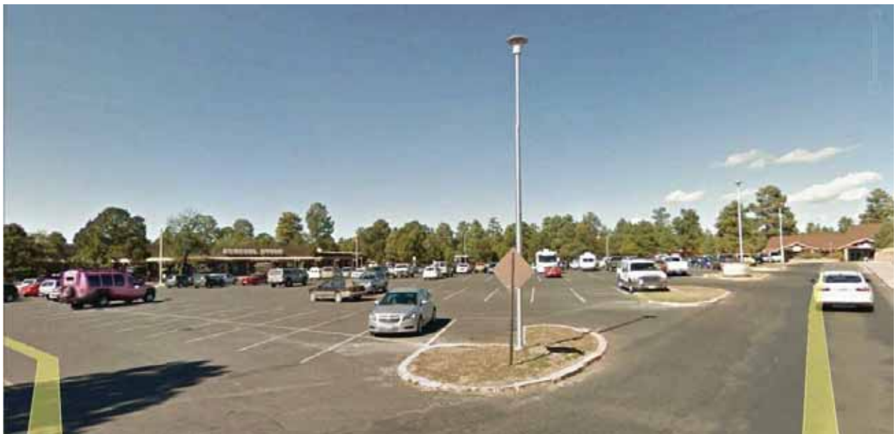
Figure 44. Pole-mounted, partly shielded area lights at Market Plaza.
