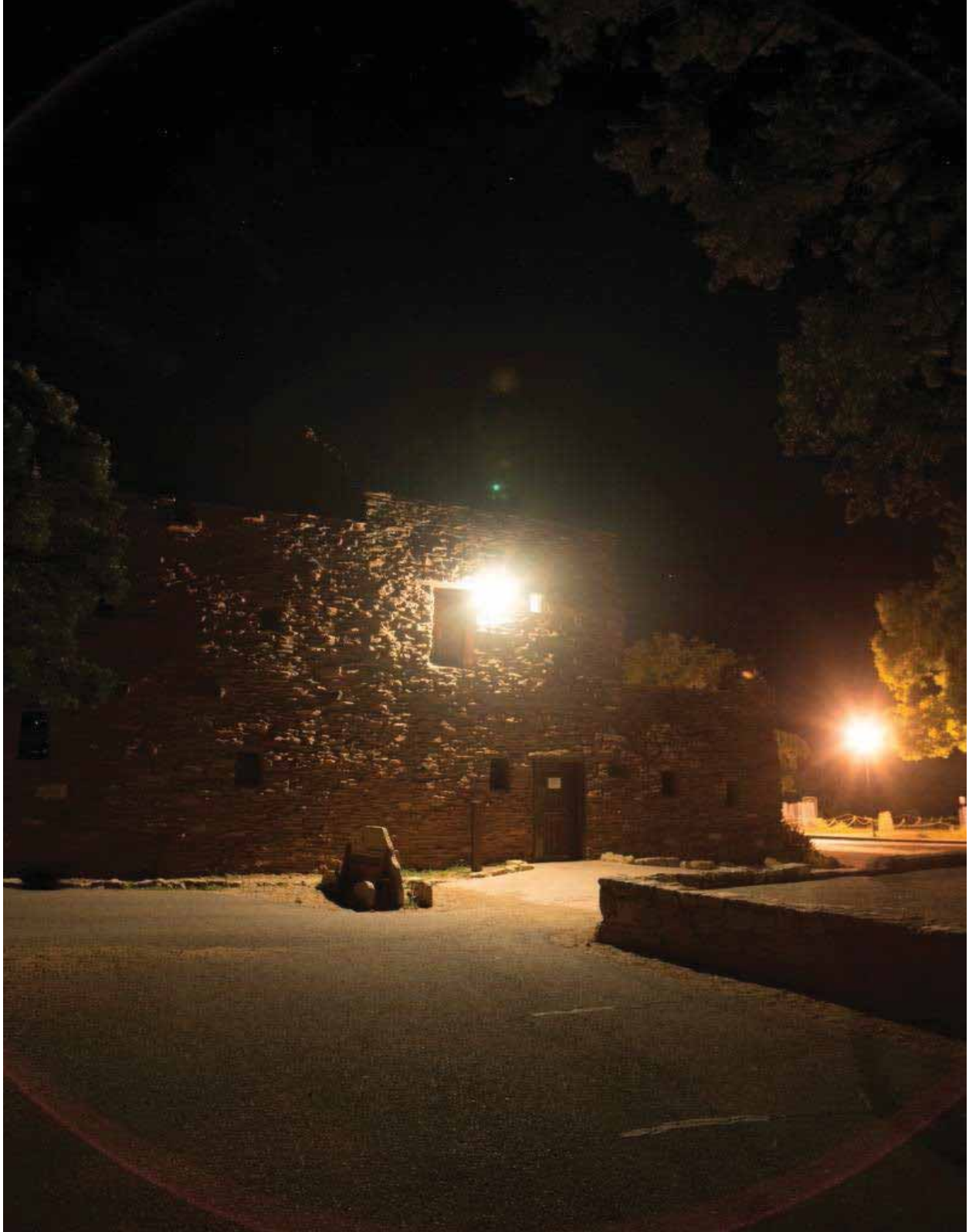
Figure 39. Horizontally aimed floodlight at Hopi House.
