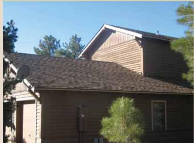
*This renovation project includes replacing windows, exterior doors, and roofs; upgrading electrical systems and plumbing; refinishing or replacing floors; repairing foundations; rodent-proofing; and installing fire sprinkler systems.*
