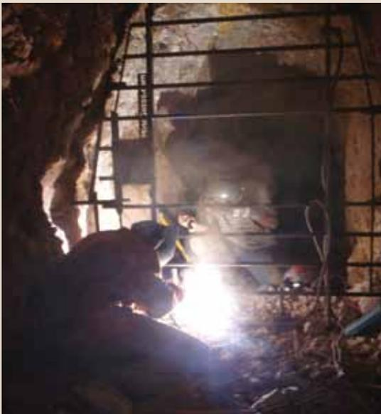
*Installation of bat gates on Horseshoe Mesa in 2009. The NPS has undertaken several projects at abandoned mines throughout Grand Canyon to seal them for the safety of park visitors. Funds from the American Recovery and Reinvestment Act of 2009 (ARRA) are being used to secure numerous mine openings at the defunct mines. Teams are installing bat gates and posting warning signs where appropriate. NPS photo*
