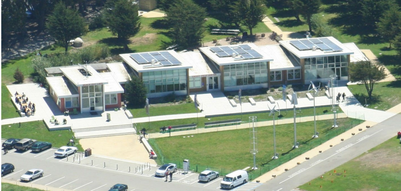
Building 1199 at Crissy Field is a LEED Platinum building occupied by GGNRA's Interpretation Staff. It features solar panels, wind turbines, rainwater catchment, daylighting, sustainable materials, and EV charging.
