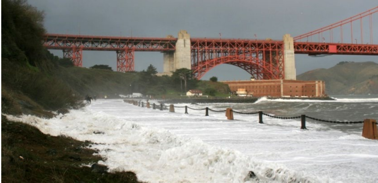
High tides and flooding wash over the entrance road to Fort Point National Historical Site.
