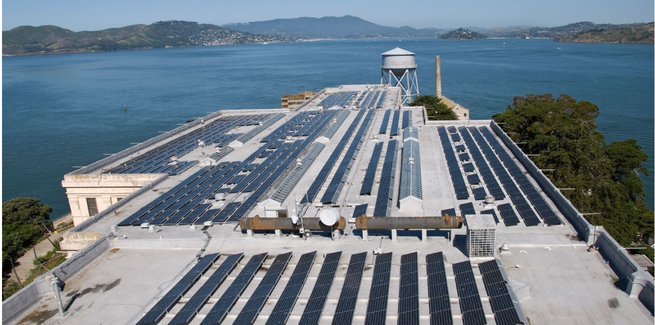
Solar panels were installed on Alcatraz Island in 2012 as part of a hybrid microgrid. The system components include solar panels, battery storage, and backup diesel generators. When functioning, the system contributes significantly to reduced park emissions, but keeping the system operational has been challenging.
