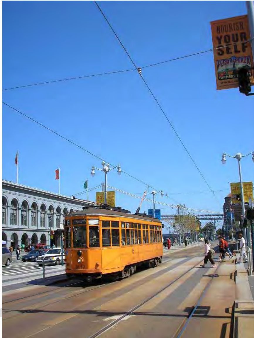
Figure 2.12.3 – Typical Double Track OCS Suspended From Span Wire (Section shown on The Embarcadero at the Ferry Building)
