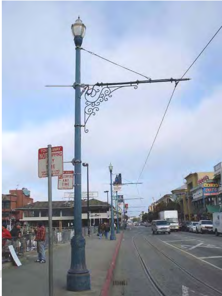
Figure 2.12.1 – Typical pole with mast arm for OCS suspension for single track (Section shown on Jefferson Street)
