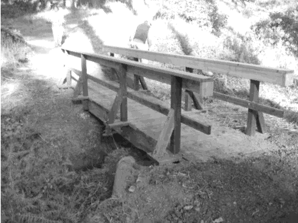
Figure 10: Typical wooden bridge and footings used to span greater than 5 foot distances.
