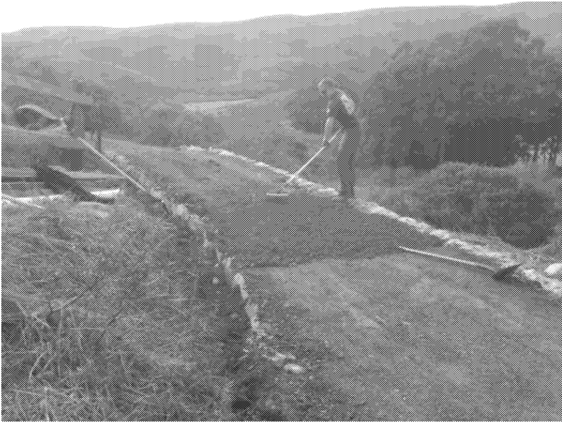
Figure 8: Typical elevated trail causeway with rock to facilitate drainage
