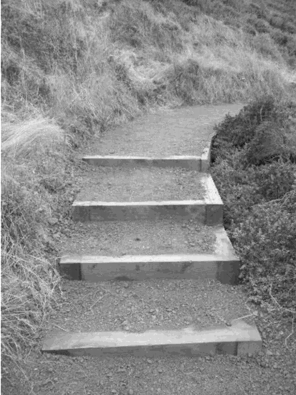
Figure 9: Typical wooden staircase (box steps)
