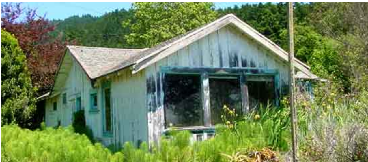
Abandoned building removal
