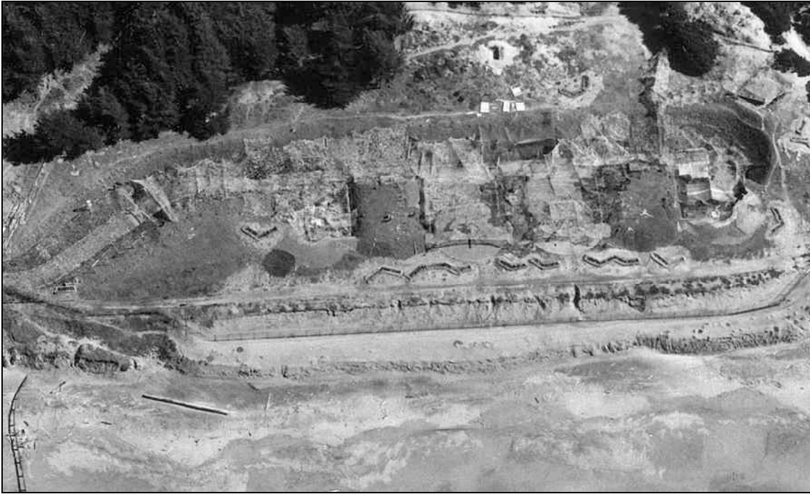
Figure 23. Battery Chamberlin in February 1942. Camouflage nets cover the gun positions and roads. The zigzag forms in front of the battery are trenches dug by the troops for close-in defense. (PARC, GOGA, Cooper Coll.)
