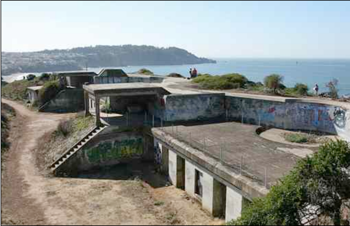
Figure 14. Battery Crosby typifies the two-story construction of an Endicott era battery. The gun was mounted in the semicircular area at right while ammunition was stored on the lower level. An ammunition hoist was located under the extended concrete canopy at center. (JAM, 2006)
