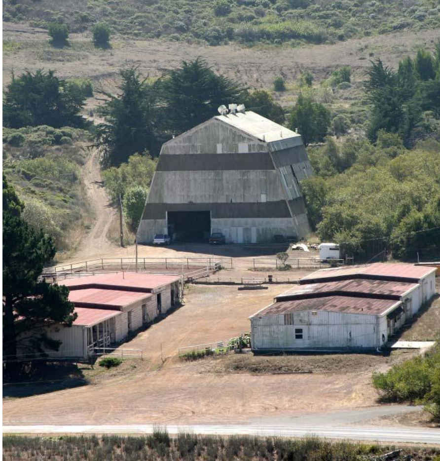
Fort Barry Balloon Hangar and Motor Vehicle Sheds, (NPS Photo, 2004)
