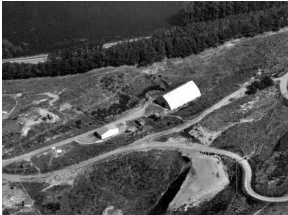
Ft. Funston Balloon Hangar, San Francisco, 1942 (now demolished). (PARC, GOGA)
