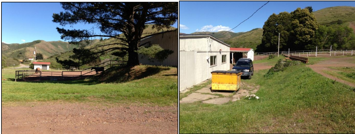
Topographic benches remain from the earliest military activity at the site and should be preserved intact.
