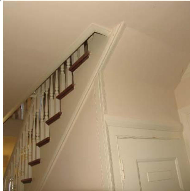
Fig. 64 :Painted wood stair, balustrade, and door at the Officer in Charge Quarters.
