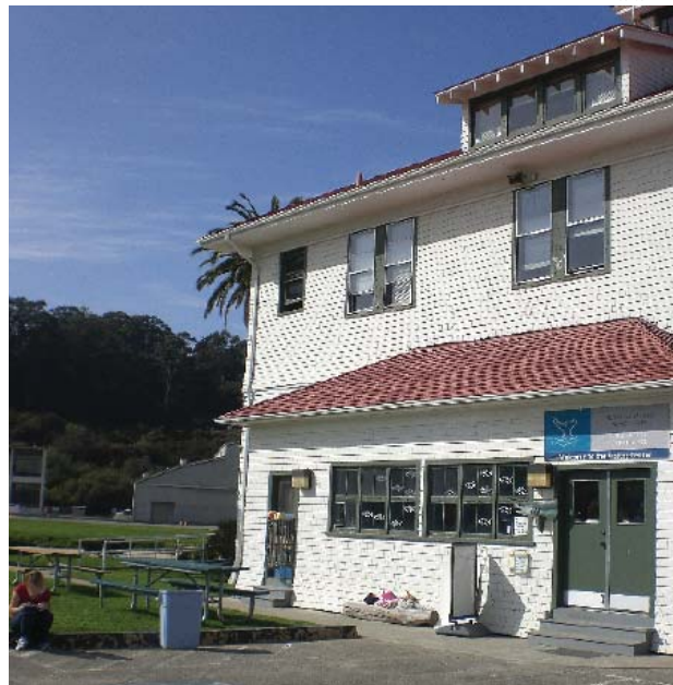
Fig. 42 : East elevation, enclosed porch of the Main Boat-house
