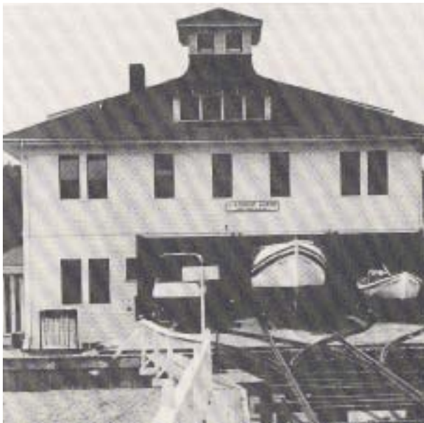
Fig. 37 : North elevation, the original window configuration of the Life Safety Station, 1919.
