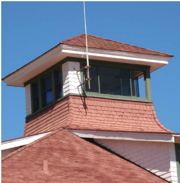
Fig. 53: Aluminum sliding window at the Main Boathouse
