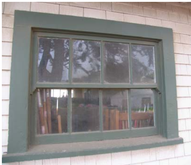
Fig. 51: Four-over-four lite windows at the Main Boathouse.
