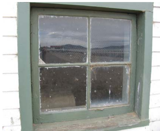
Fig. 52: Four-lite awning window at the Shop & Garage.
