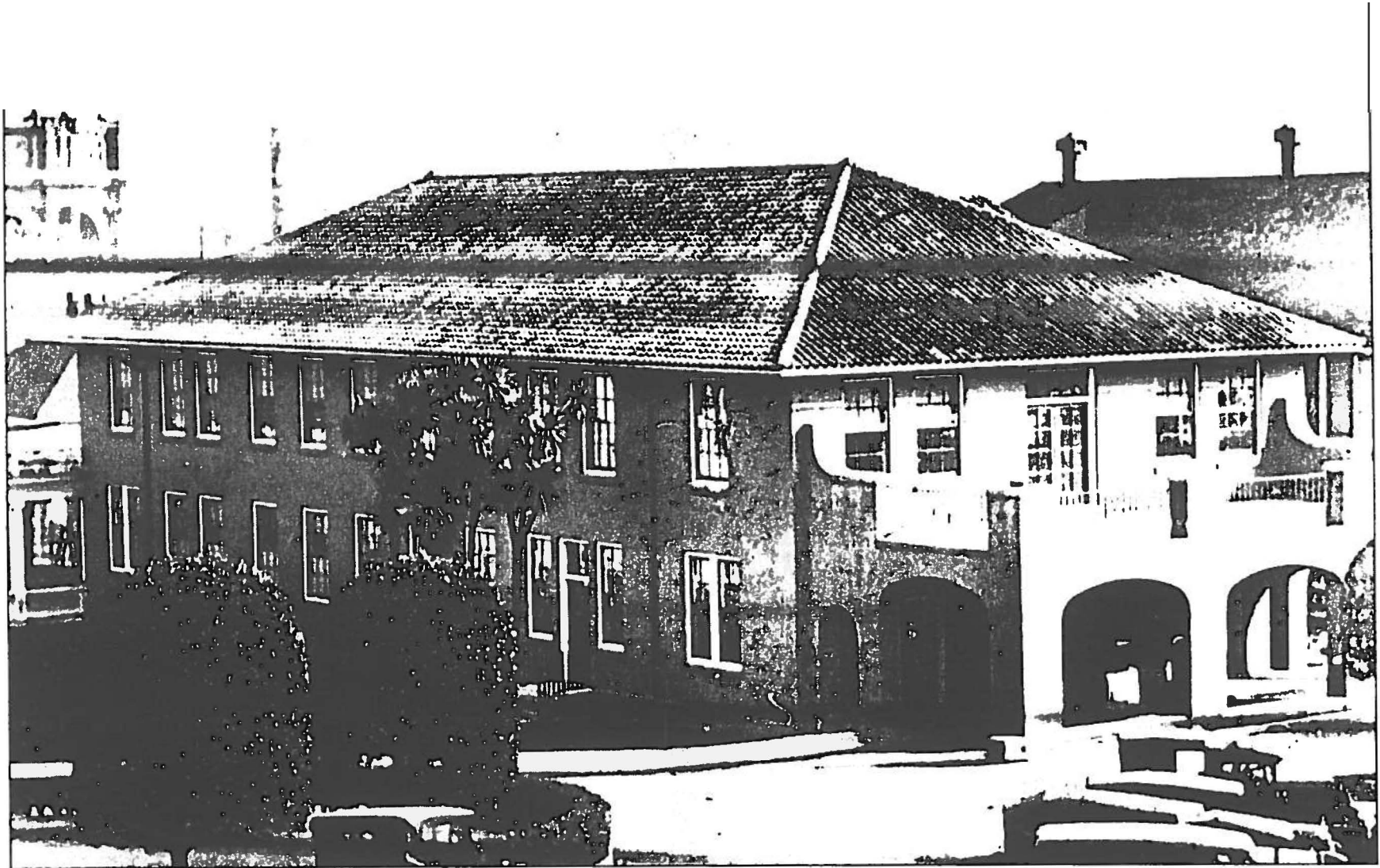
Building 1014, a receiving ward and clinic built in 1924, follows the Spanish Mission Revival tradition in Presidio architecture, while presenting a feeling of massive simplicity and horizontality. Note the enclosed gallery connecting it to the adjacent structures, and the Palace of Fine Arts in the background.
