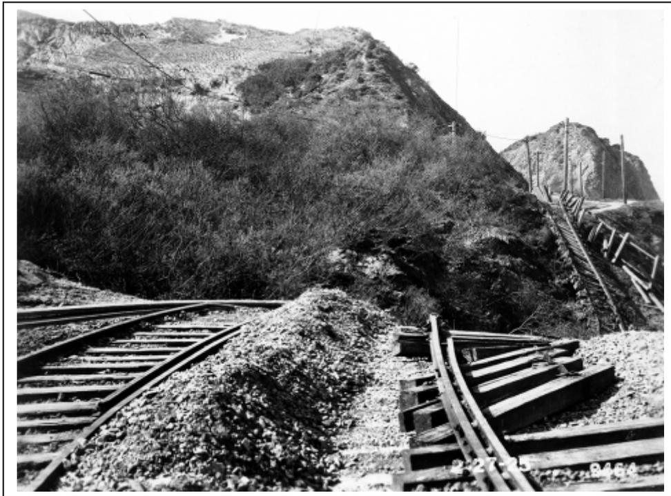
*Figure 26. A view taken in February 1925 showing one of the slides that closed the cliff line. The hillside cut in the background marks the former site of the west railroad tunnel. (John Gerrard Graham Collection)*
