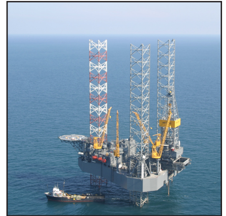
Gulf of Mexico off shore drill rig (Credit: MMS)
