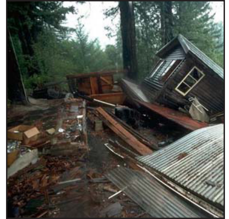
Loma Prieta earthquake
