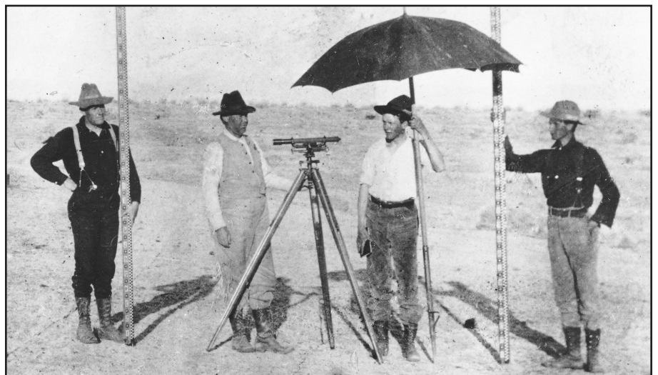
Leveling crew 1905 Keeler, CA (Credit: USGS)
