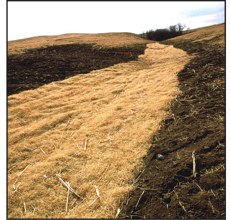
Erosion control with fiber netting
