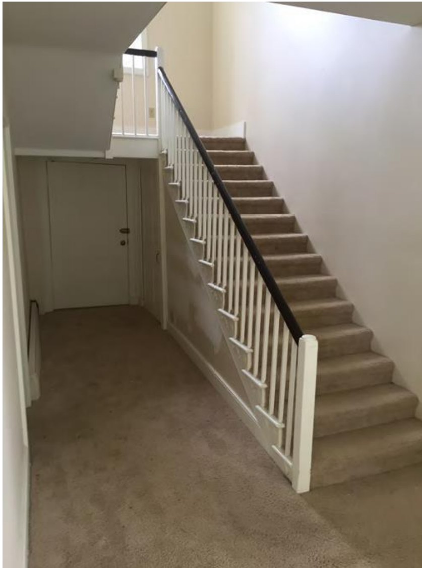
Figure 9. Entrance hall and staircase to second floor. This hall maintains original historic layout and staircase, concealed wood plank floor, and doors are considered historic features, to be preserved in rehabilitation.
