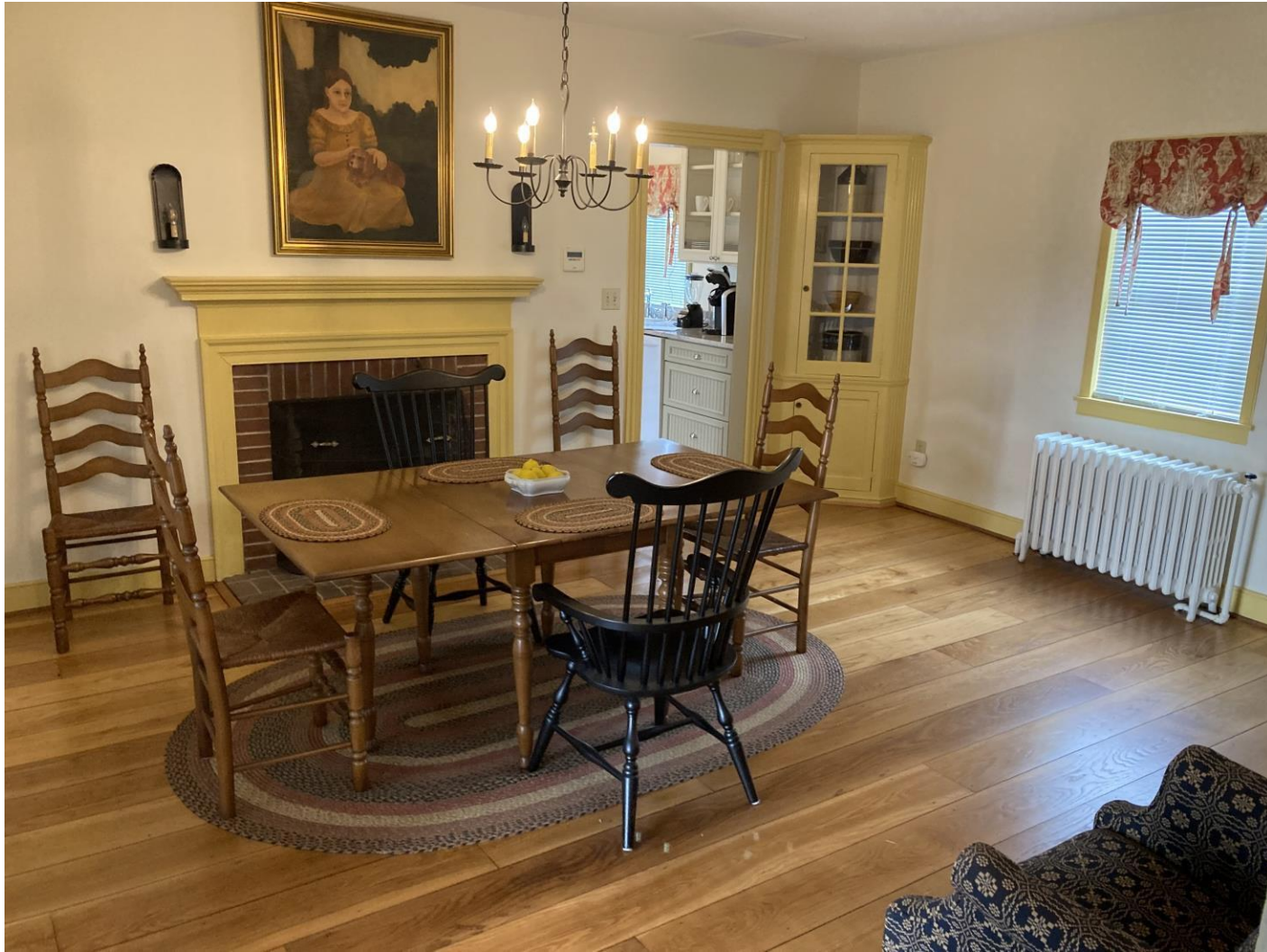
Figure 8. Dining room, rehabilitated 2017 and carefully furnished and decorated with a period theme. Historic features include the brick hearth and fireplace mantel, door and window casings and beaded molding, built-in corner cupboard. Modern tongue and groove wood flooring reflects the original floor material.
