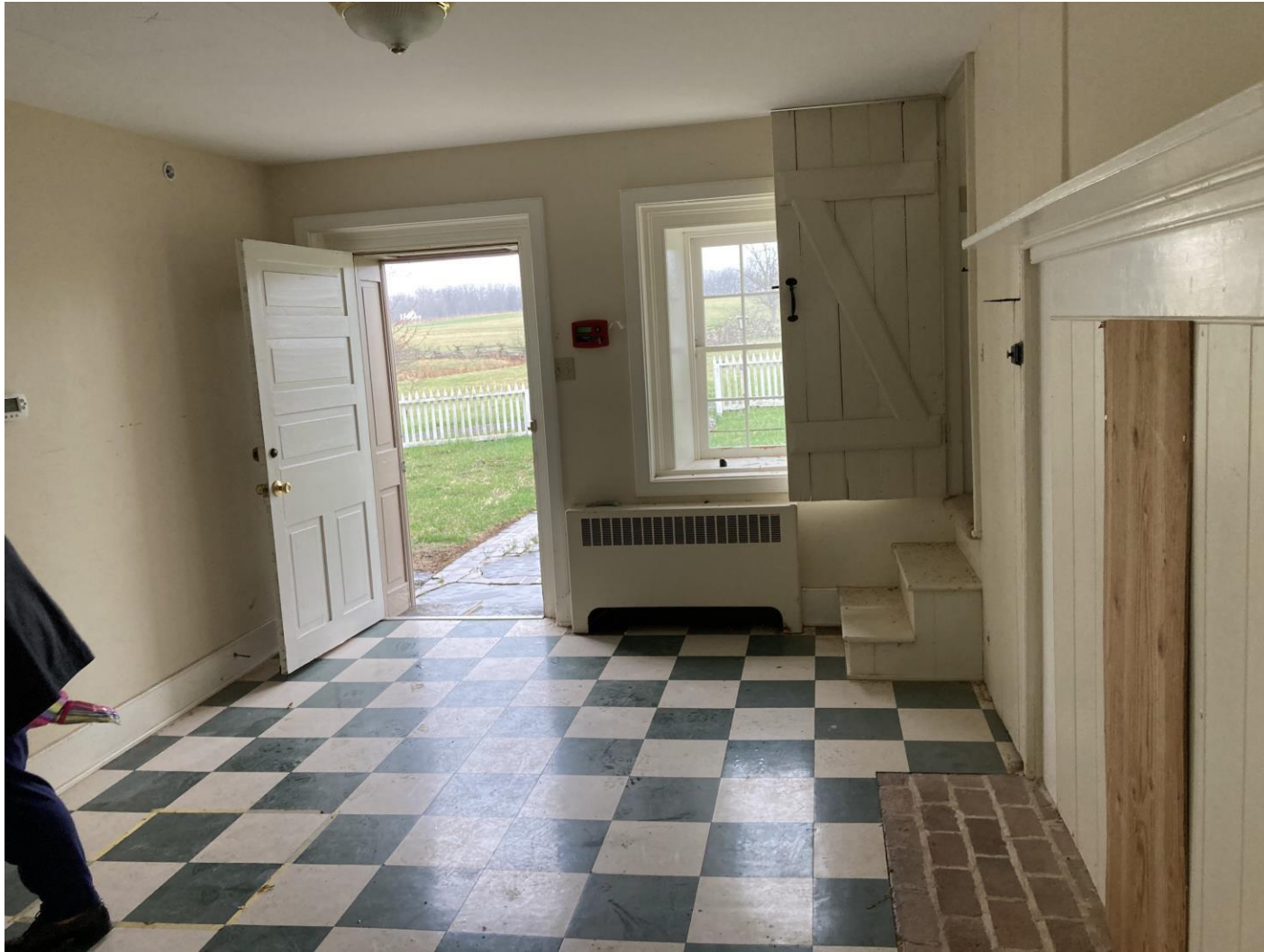
Figure 5. Rose Farmhouse, laundry (proposed sitting room), first floor addition. Note enclosed historic firebox, some original plaster on walls, 1980s vinyl floor and furred out exterior wall. This room is adjacent to the kitchen and pantry (proposed bathroom). Stairs visible on the right access the second-floor bedroom
