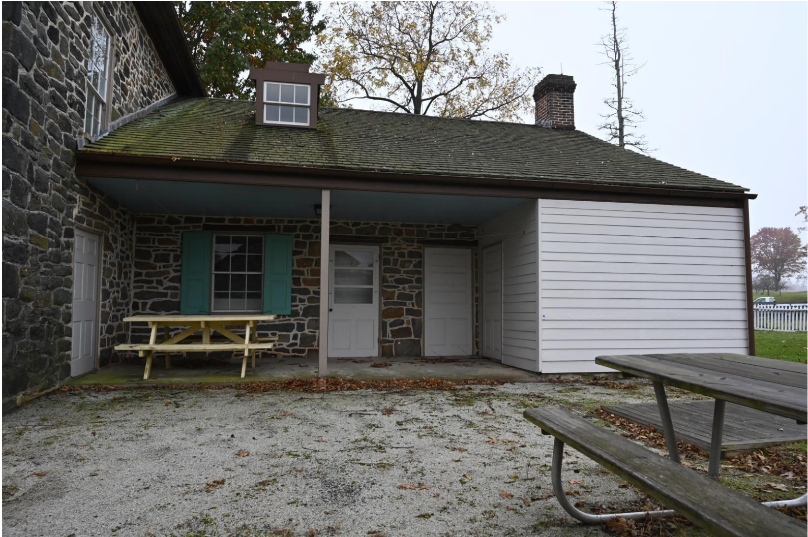
Figure 7. Rose Farmhouse, rear patio off kitchen, east elevation. A brick patio previously extended from the concrete. The horizontal wood siding addition is the previous pantry (proposed bathroom).
