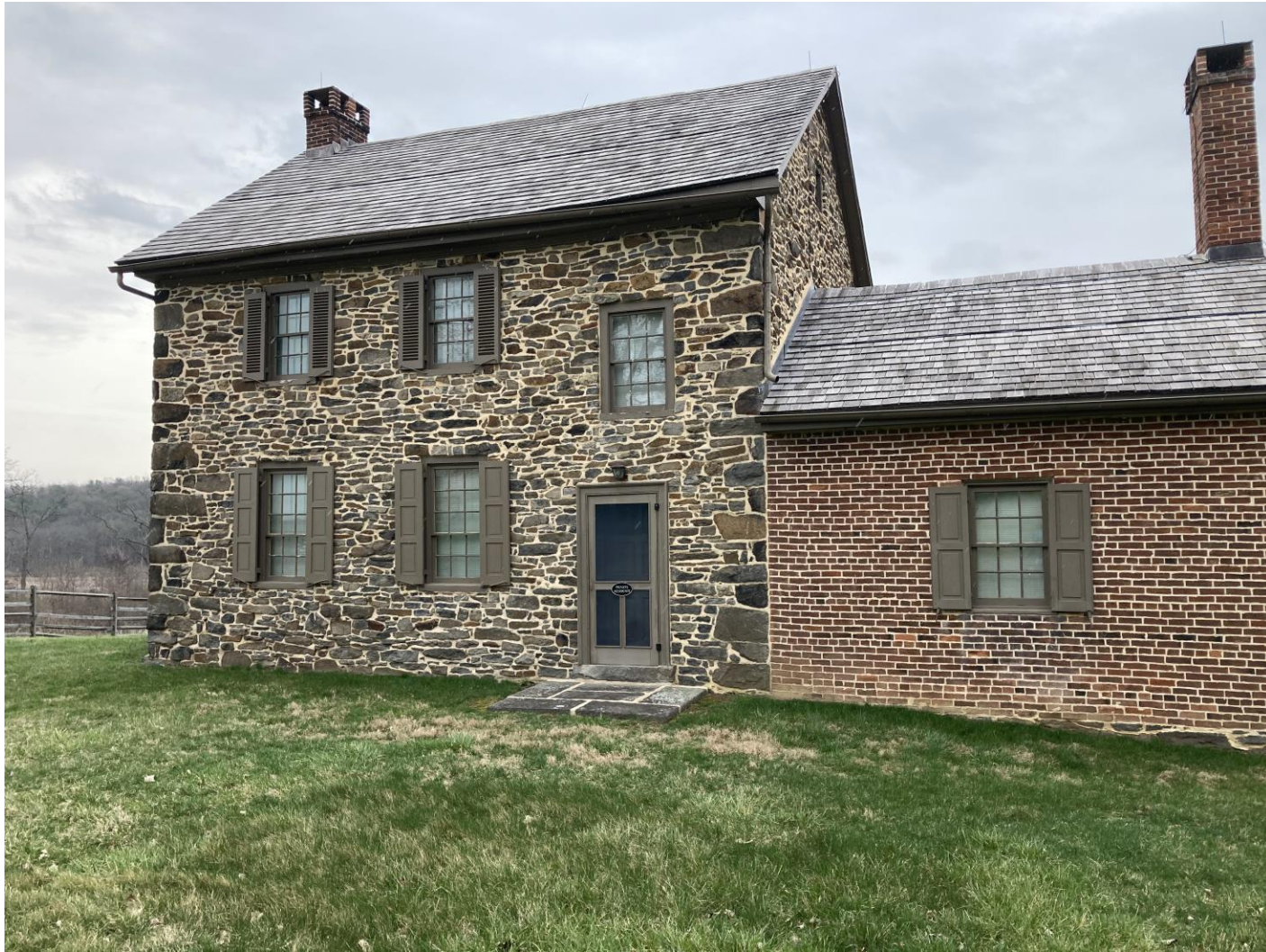
Figure 3. Bushman Farmhouse, west elevation. The original two-story native stone house on the left dates to ca. 1808, with oversize cut stone quoins ( right ) and original window and door configuration. The brick addition on the right dates to ca. 1860. The combination of stone and brick is unique among Civil War houses on the battlefield. Log smokehouse, painted white (now wellhouse), ca. 1808.
