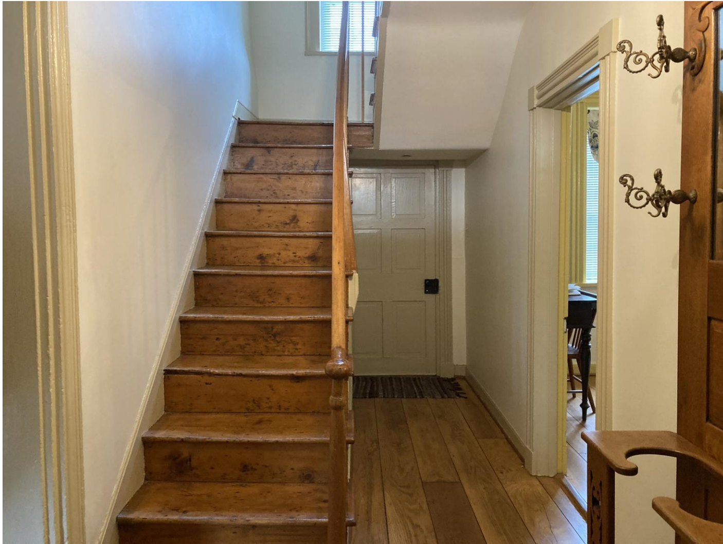
Figure 10. Central hall with original preserved staircase. While poor condition required installation of compatible material for flooring throughout the first floor in recent rehabilitation, the National Park Service was able to restore the original wood flooring in the staircase and on the second floor.
