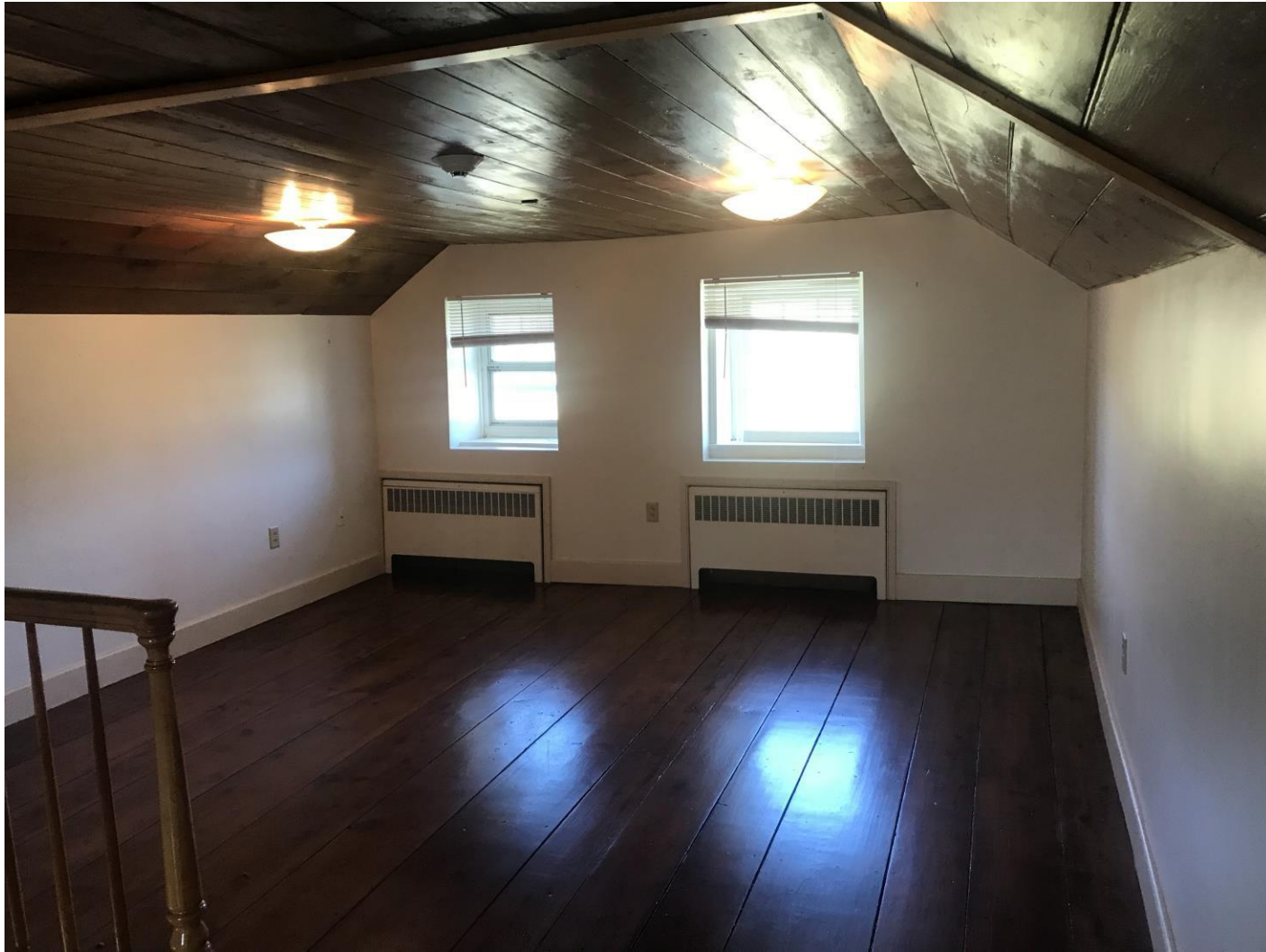
Figure 9. The open second floor bedroom of the Slyder house. Historic fabric consists of wood plank flooring and tongue and groove board ceiling.
