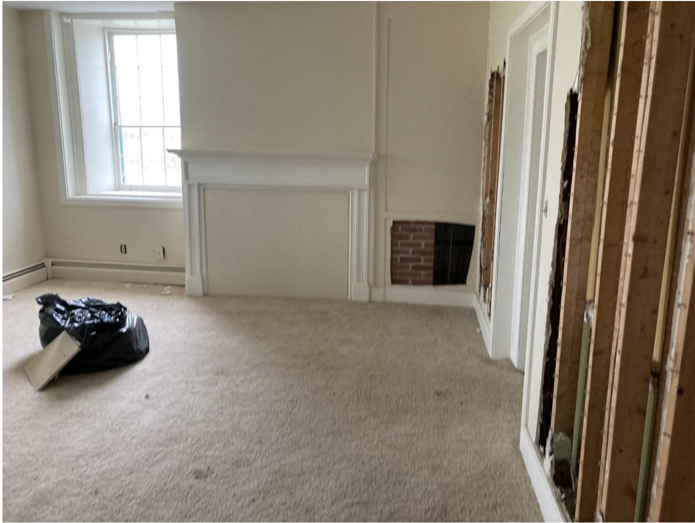
Figure 8. Rose Farmhouse, first floor parlor room. Proposed rehabilitation will return this room to intact original plaster walls (intact behind furred out walls), wood plank flooring, brick firebox and hearth.
