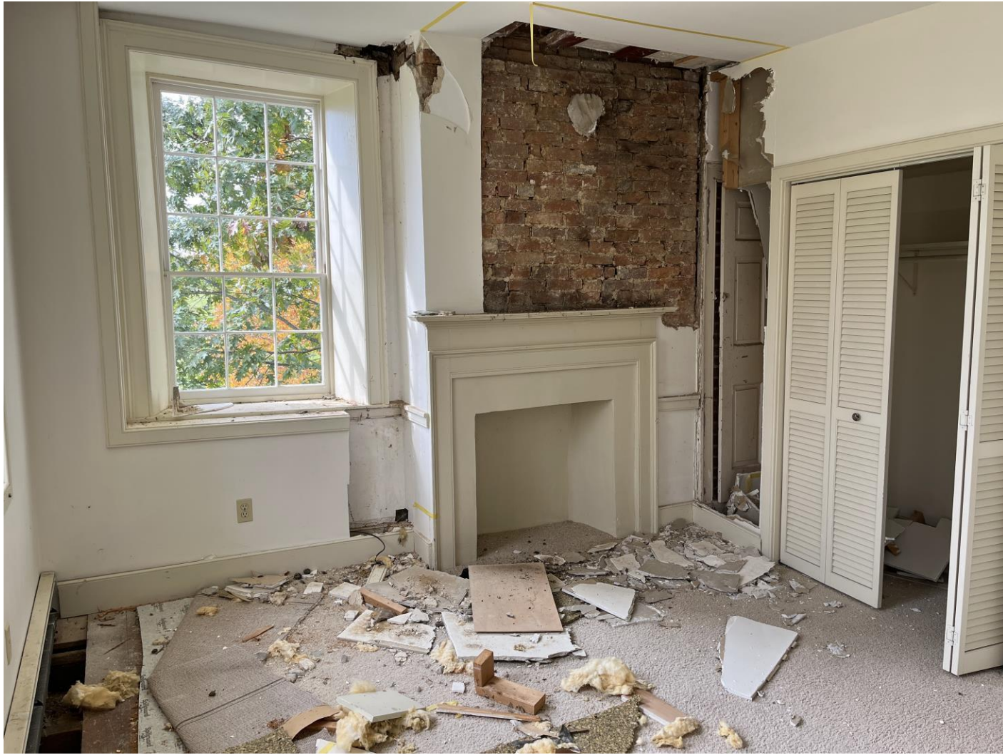
Figure 10. Bedroom #1, second floor. Walls and floor opened to expose historic fabric to help inform rehabilitation.
