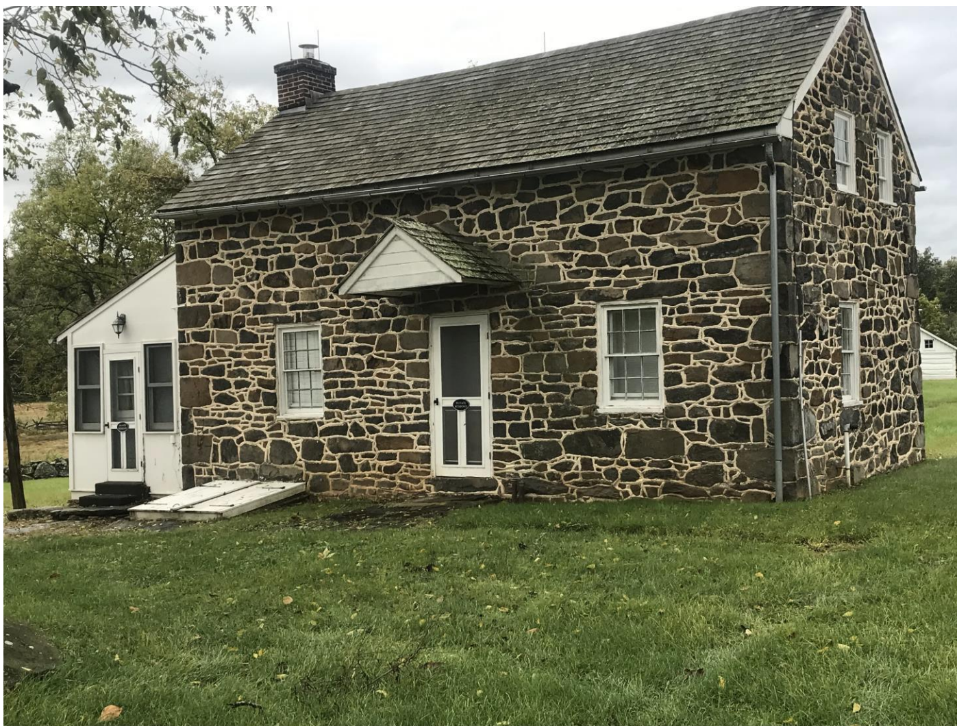
Figure 2. Two-bay, two story Slyder Farmhouse, south elevation. A two-story, two bay house with native stone exterior walls and rough-cut diabase stone wall edges. A non-historic frame addition on the west end includes sunporch and bathroom.
