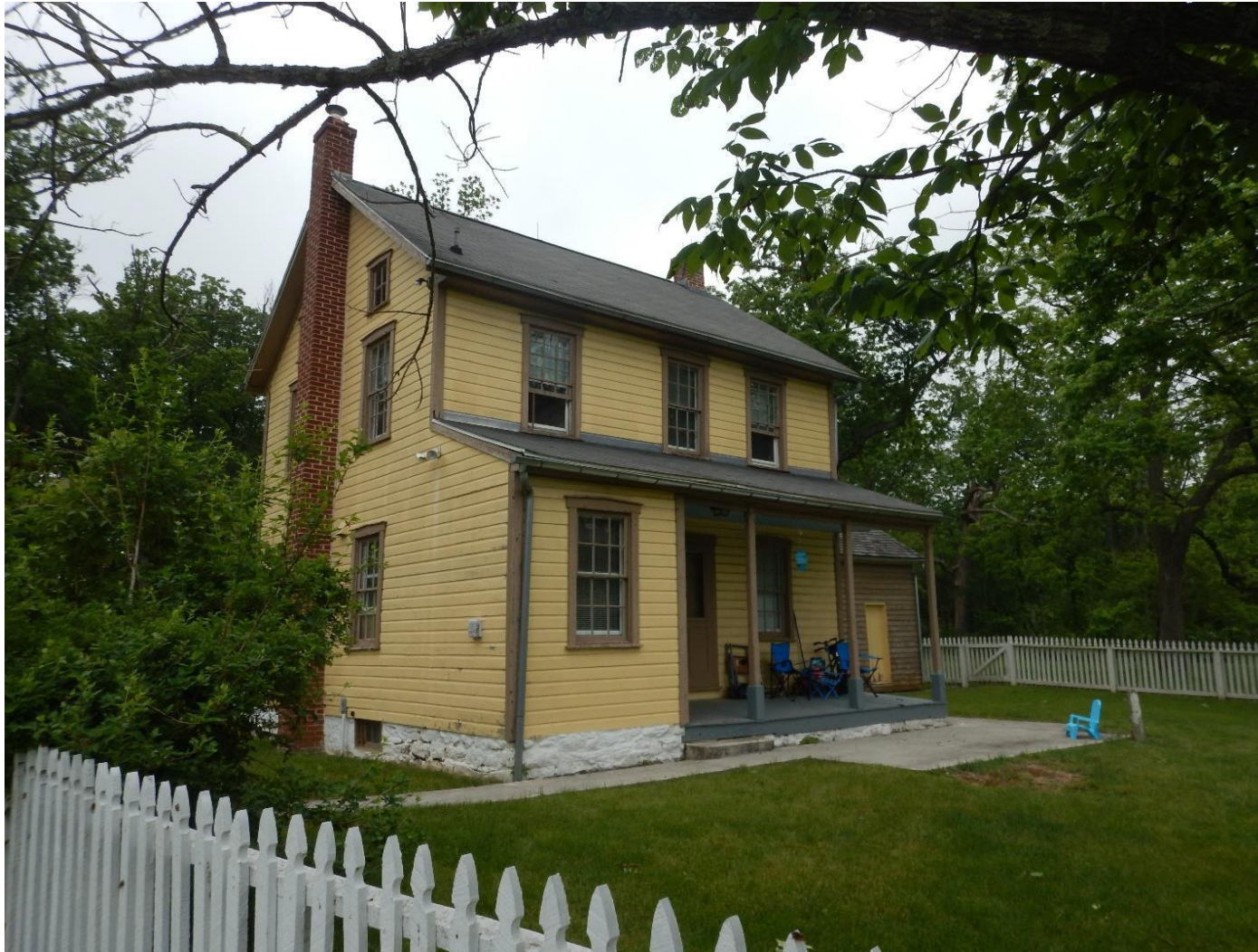
Figure 3. Front (south) and west elevations of the Althoff Farmhouse. The drop siding exterior, overall arrangement of windows and doors, and window type (divided light, wood double-hung) are considered historic features.
