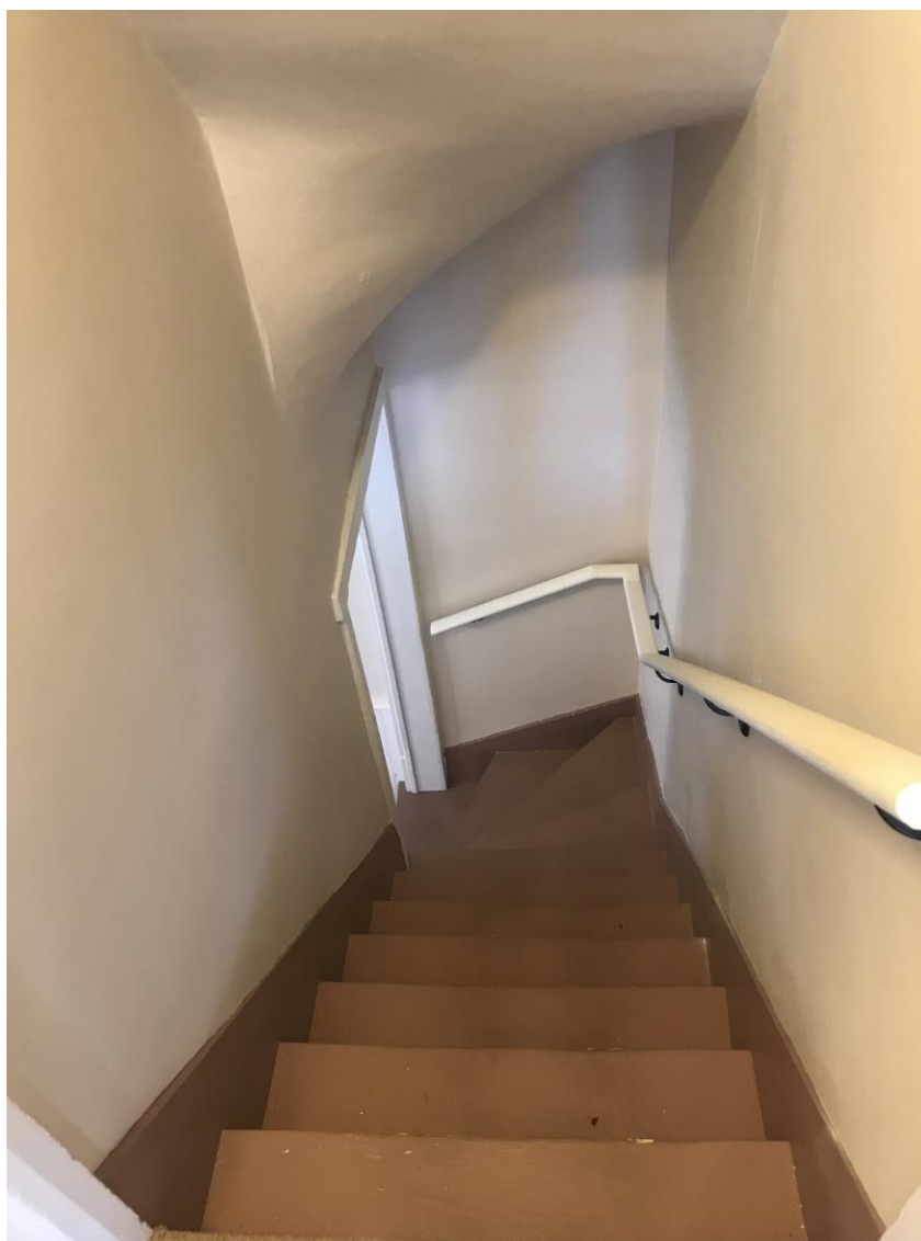
Figure 12. Kite winder staircase, a key historic feature.
