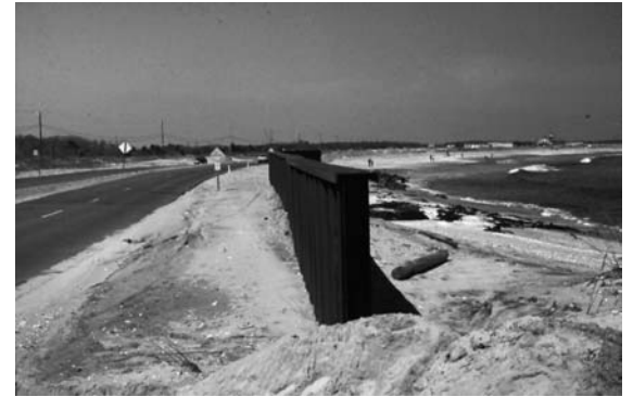
Steel Wall at the Critical Zone
