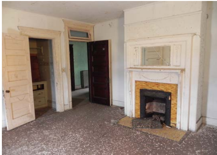
Building 6 bedroom, second floor. NPS PHOTO
