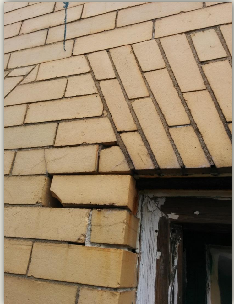
Building 7 Exterior - Loose Bricks Around Window
