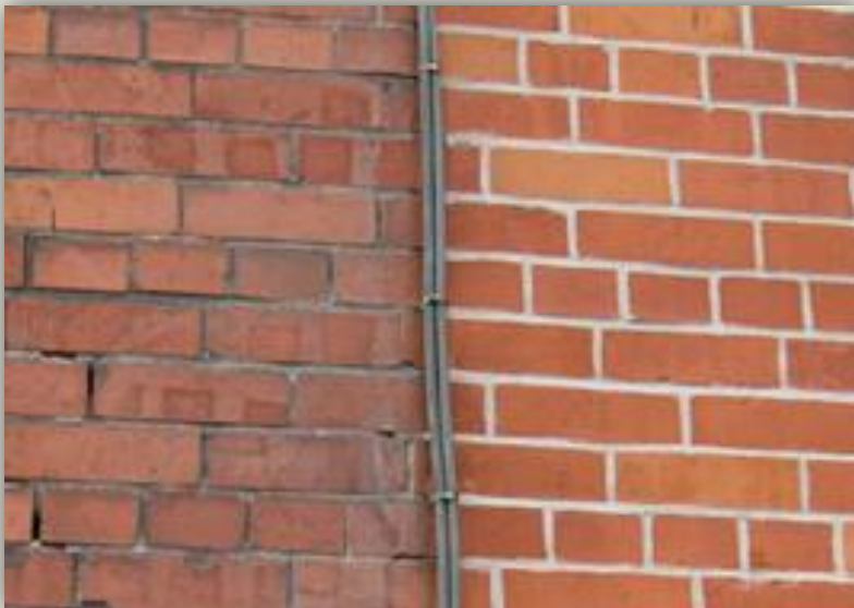
Example of Brick Repointing Before + After
