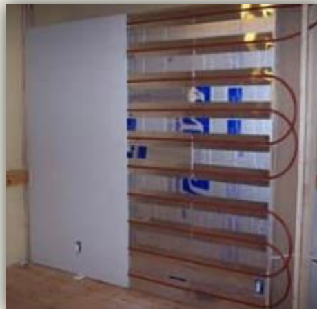
Example of PEX Wall Radiator
