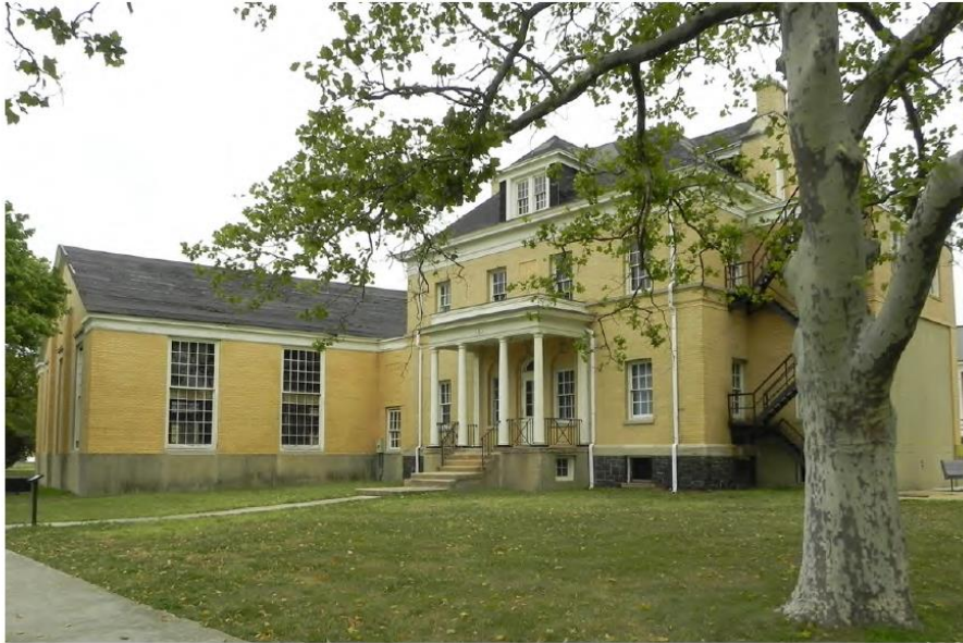
RIGHT: Building 40, former YMCA, showing both the front entrance and the basketball court extending forward. NPS PHOTO
