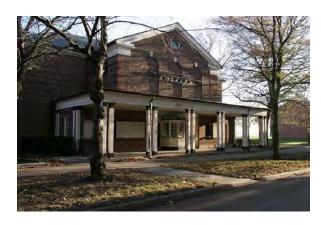
**Building 330** is a 700-seat theater with a stage and projection screen, built in 1937. The charming ticket booth, curving entrance ramps and theater area are all in excellent shape. The building has a cast-in-place concrete slab on grade system with cast-in-place concrete footings under load-bearing brick columns and walls. The slate roof is recently renovated.
