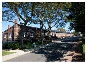
**Building 110** was constructed in 1879 and enjoys unmatched views of lower Manhattan from its lengthy northern façade. The building has brick on masonry bearing wall construction and much of the interior has wood columns at 12' spacing. New HVAC and fire suppression systems were recently installed through most of the building and a new roof is being installed. Building 110 is directly adjacent to Soissons Landing. A portion of the upper floor is currently in use for artists' workspaces.
