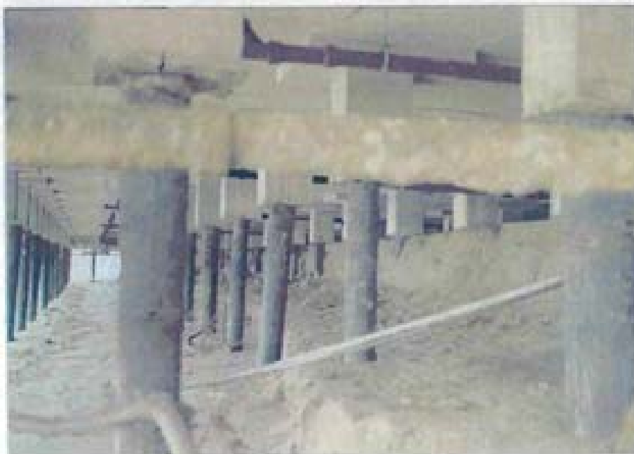
PHOTO NO. 5 ELECTRICAL CONDUIT LYING ON UNDERMINED BEACH AREA - A RESULT OF BROKEN HANGARS.
