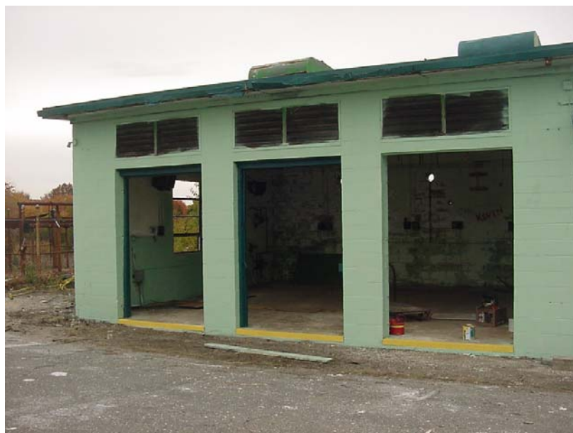
Fort Hancock Generator Building in 2003.
