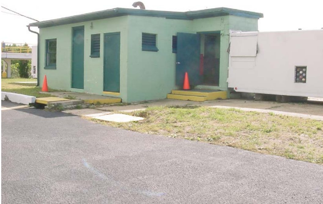
Radar vans and Inter-connecting Corridor Building in 2003.
