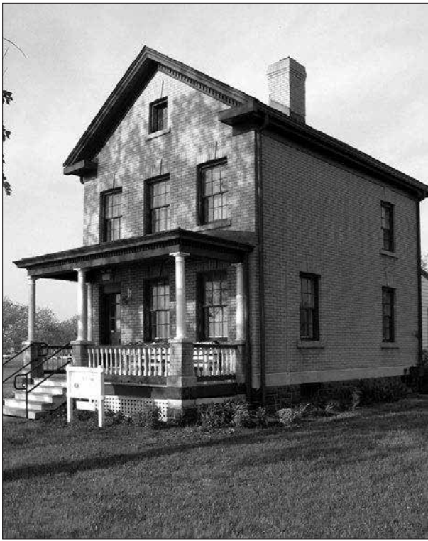
Figure 2.5. The building currently leased by the Audubon Society is typical of the smaller single family homes at Fort Hancock. OCLP, 2004.
