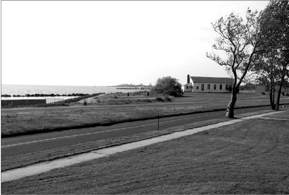
Figure 2.8. Poured concrete sidewalks line the east side of Hartshorne Drive. OCLP, 2004.
