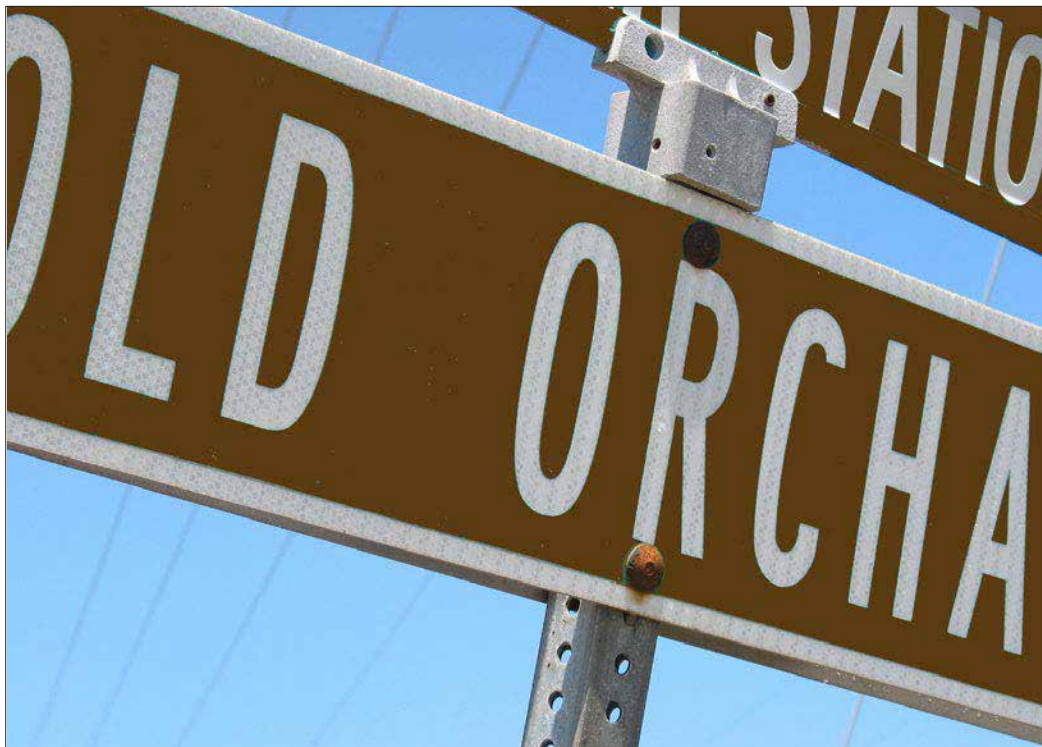
Figure 2.38. This street sign from off-site shows the mounting hardware and configuration of the recommended street signs for Fort Hancock. The small sign on top should be constant on all signs, reading "Fort Hancock." Lower sign panels would list street names. Brown backgrounds with white lettering is recommended. OCLP, 2005.
