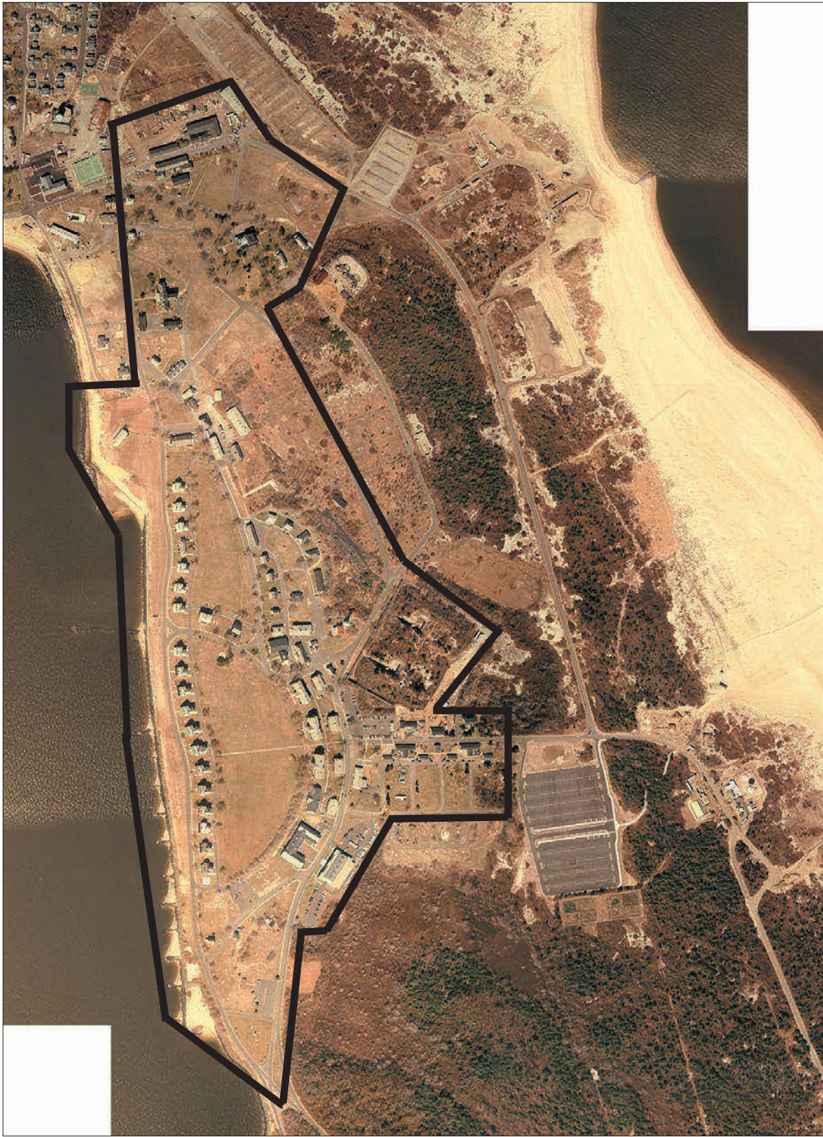
Figure 1.4. 2004 aerial photograph of Fort Hancock, Sandy Hook Unit of Gateway National Recreation Area. The study area is outlined in black. GATE files.
