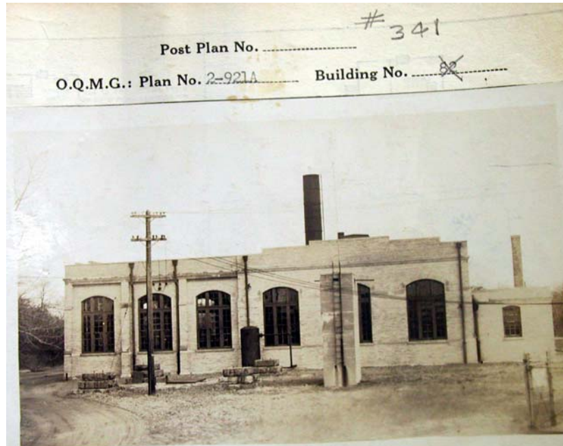
Fort Hancock Pumping Station Photos courtesy of NPS/Gateway NRA
