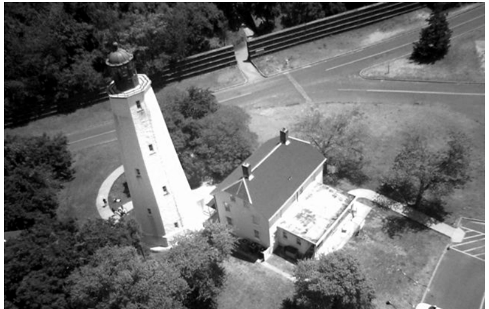
Sandy Hook Lighthouse & Keepers Quarters, located in the Fort Hancock area of the park.
