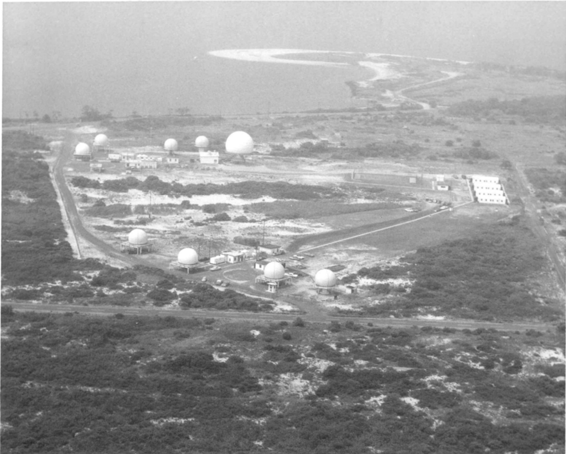
Fort Hancock's Nike Integrated Fire Control (IFC) Area. Photo courtesy of NPS/Gateway NRA
