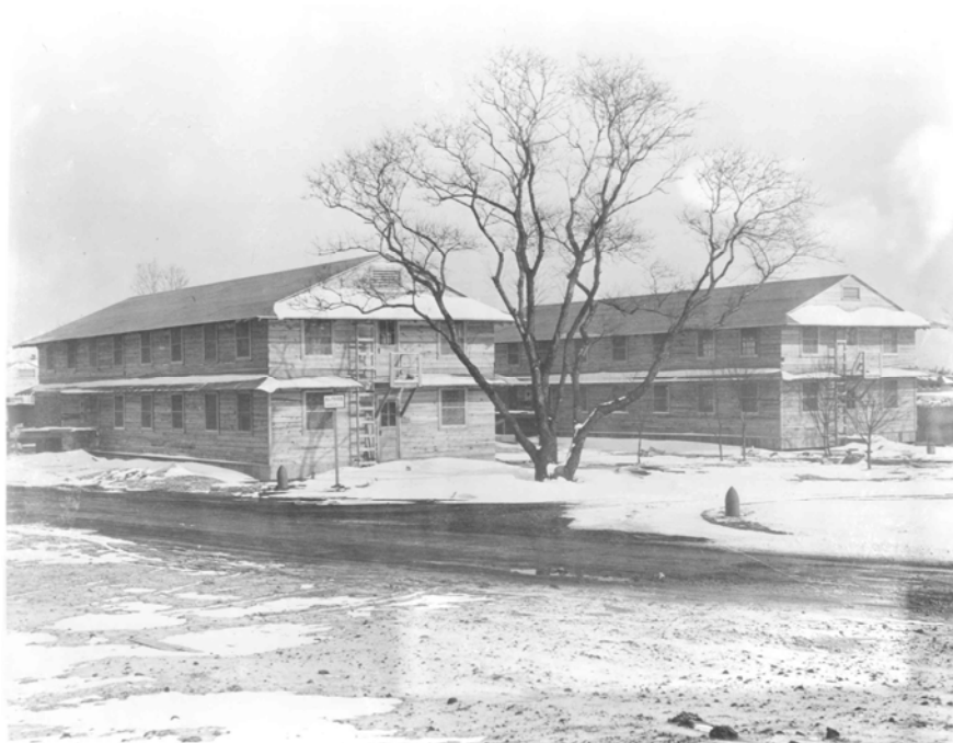
Temporary Barracks at Fort Hancock to house the influx of soldiers during World War II. Photos courtesy of NPS/Gateway NRA
