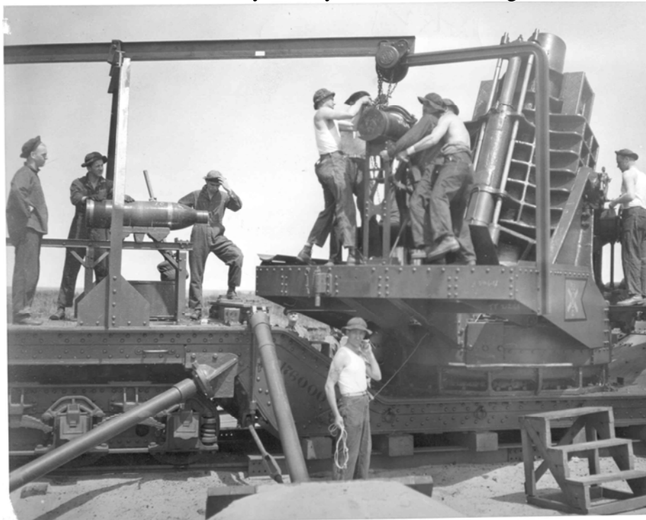
12 inch mortar being loaded
