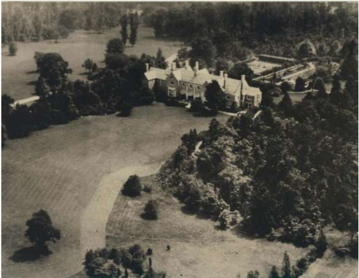
40. 16-29 ALDRED, Lattingtown / Glen Cove, Long Island, NY ("Ormston")
