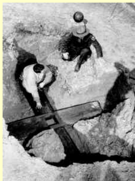
1958 Excavation - 1814 flagstaff cross brace timbers
