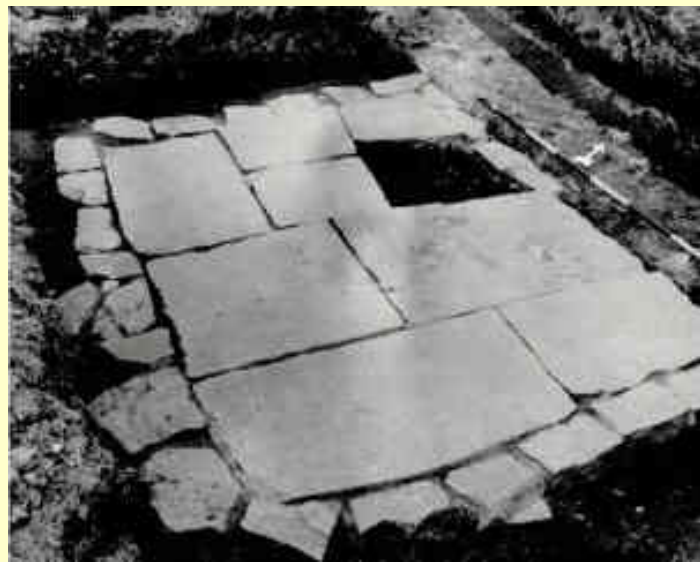
Stone slab foundation - 1776 Powder Magazine
