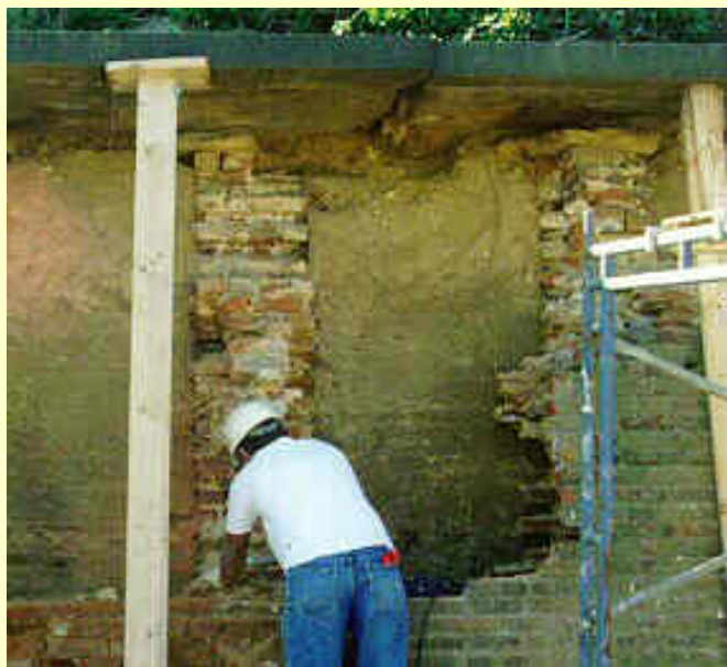
1997 Fort Wall Excavation
