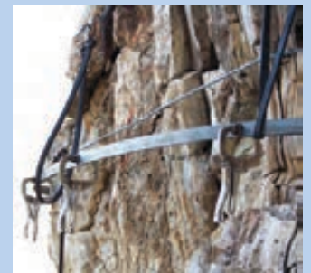
Metal bands are installed around cracked stumps.
