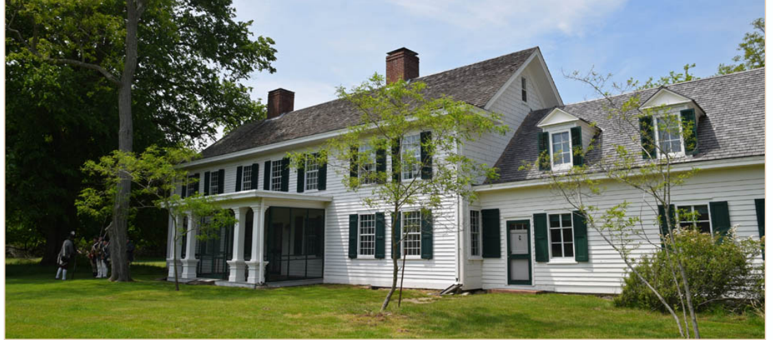
Among the climate impacts of greatest concern to the William Floyd Estate are strong winds and stronger storms—such as Nor'easters and hurricanes—which cause damage to structures and the landscape. NPS Photo.
