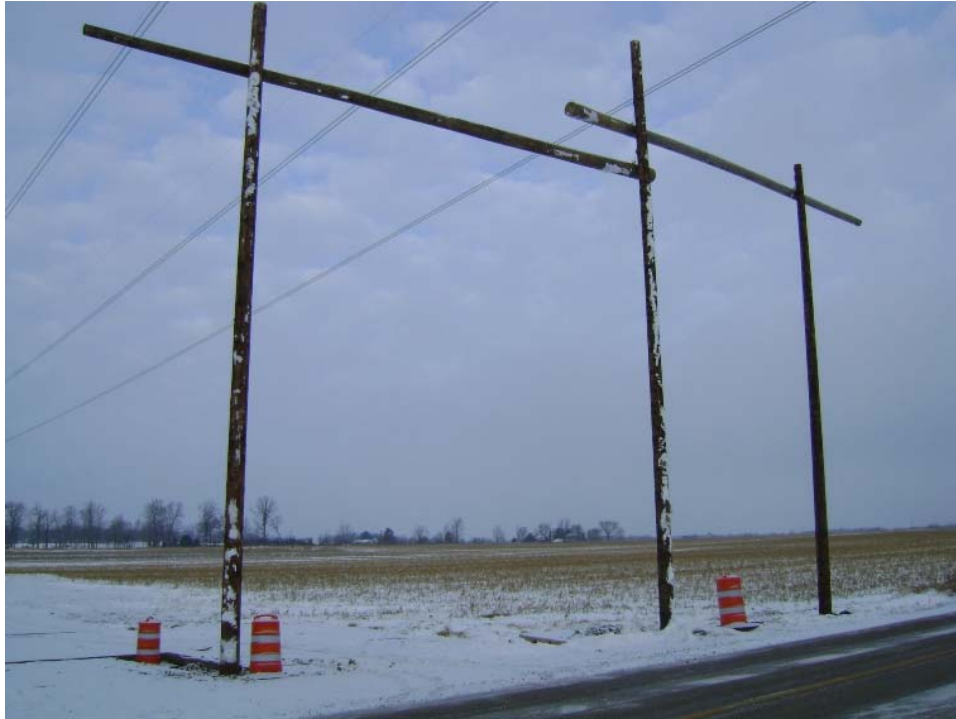
This photo is an example of the guard structures for stringing conductors during construction.
