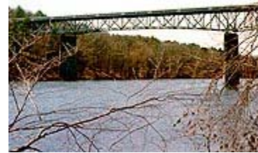
Milford-Montague Bridge today.
