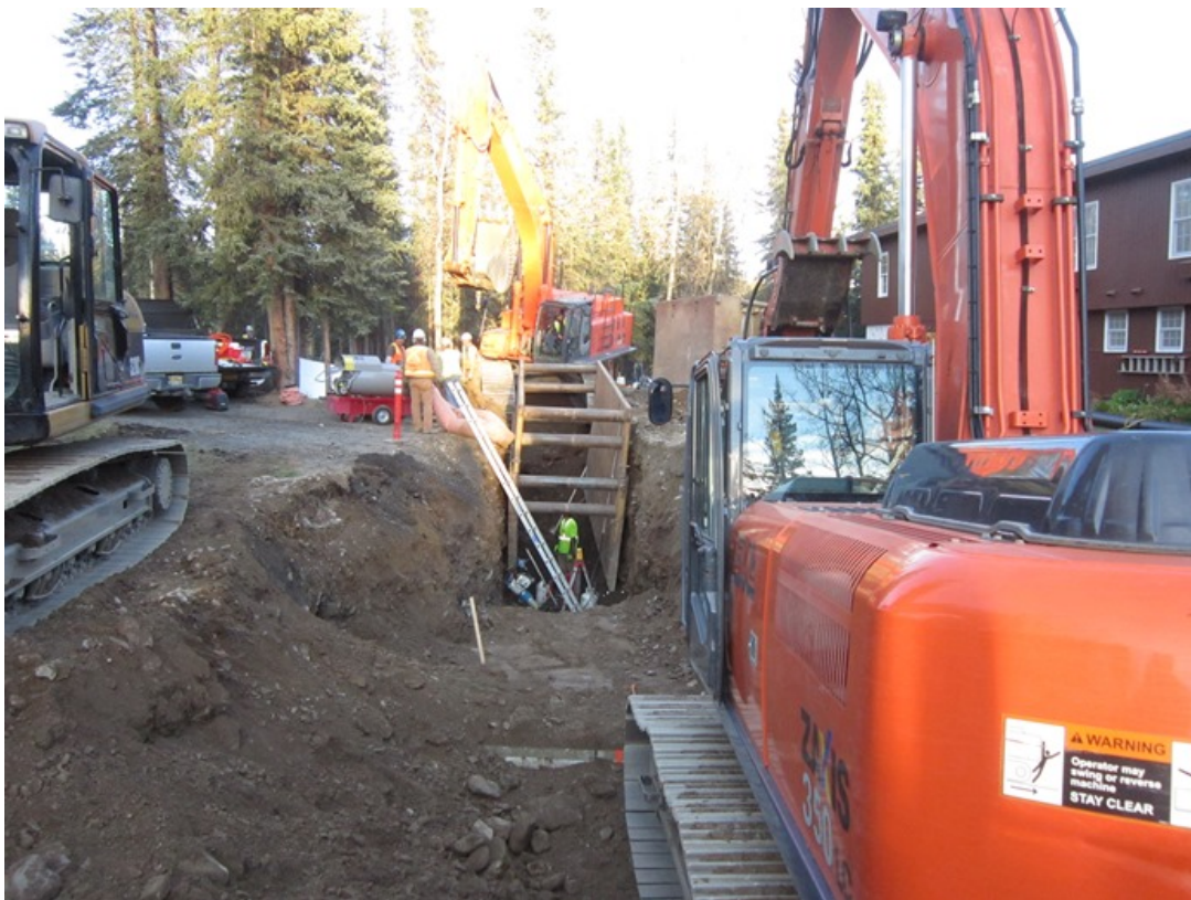
Utilidor replacement in park housing area
