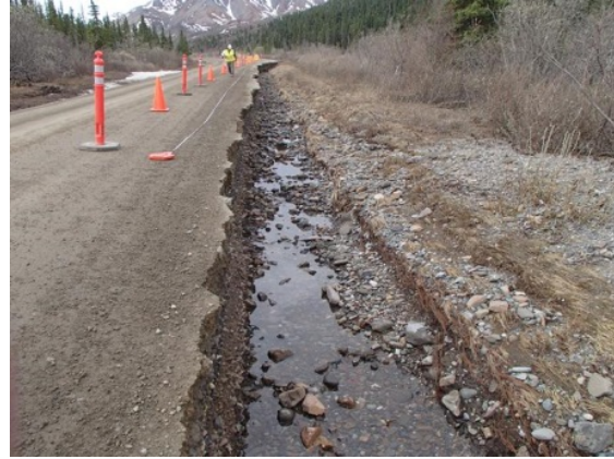
Raging current tearing at park road at Mile 20-22 and resulting damage
