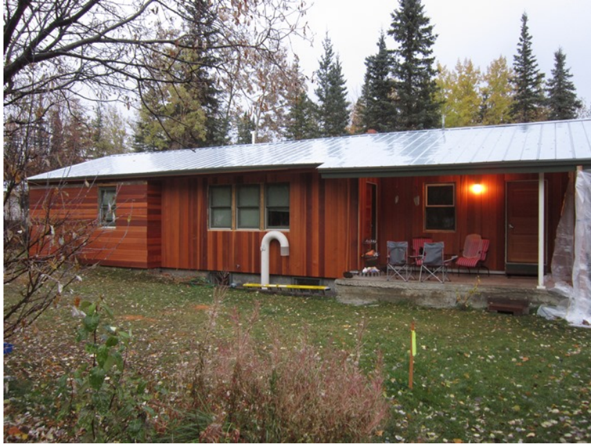
Restored Quarters P26
