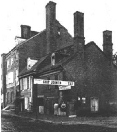
The pole gutters on the roof at 757 Swanson Street, Philadelphia in 1868 divert rainwater to a short cylindrical downspout. Moisture damage is evident on the wall of the building below the end of the pipe where there is no downspout extension. (Print & Picture Collection, The Free Library of Philadelphia) [click image for larger view]
