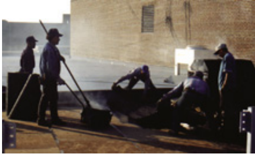
The first ply of hot applied, built-up roofing is installed over perlite insulation board. The system is carefully installed to accommodate locations of roof penetrations and rooftop mechanical equipment. (Photograph courtesy of Wiss, Janney Elstner and Associates)
