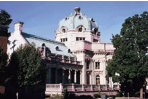
Copper was put to effective use on the roof of the 1913 Handley Library in Winchester, Virginia. (NPS photo) [click image for larger view]
