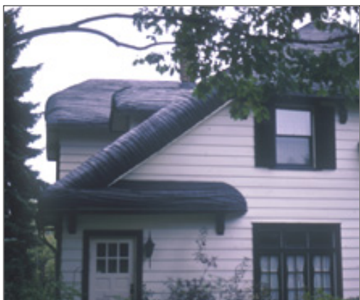
The wood shingles on the roof of this Tudor Revival house (left) were steamed and bent to resemble thatching. To aid architects and contractors to lay such special effects shingles properly, manufacturers like the Creo-Dipt Company, Inc. of North Tonawanda, New York, published roof details, like those in the 1923 Sweet's Architectural Catalogue (below). (Photograph courtesy of NPS; "Country Cottage Roof".) [click image for larger view]
