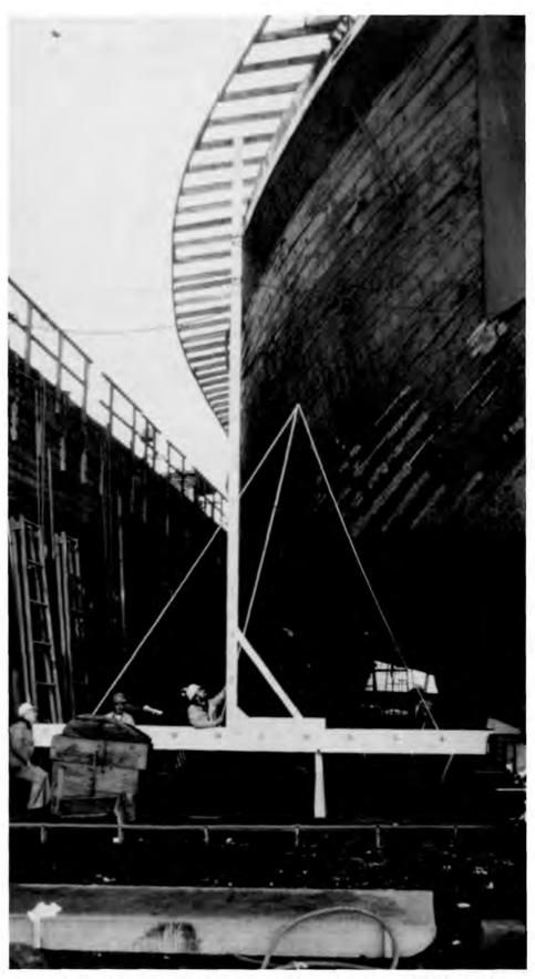
Lines-lifting team measuring points on a section plane at Wawona's bow, October 1985. Procedure required the use of two tape measures and the erection of very large squares and a straightedge specially built for the project. (Photo by Richard K. Anderson, Jr., HAER 1985.)
